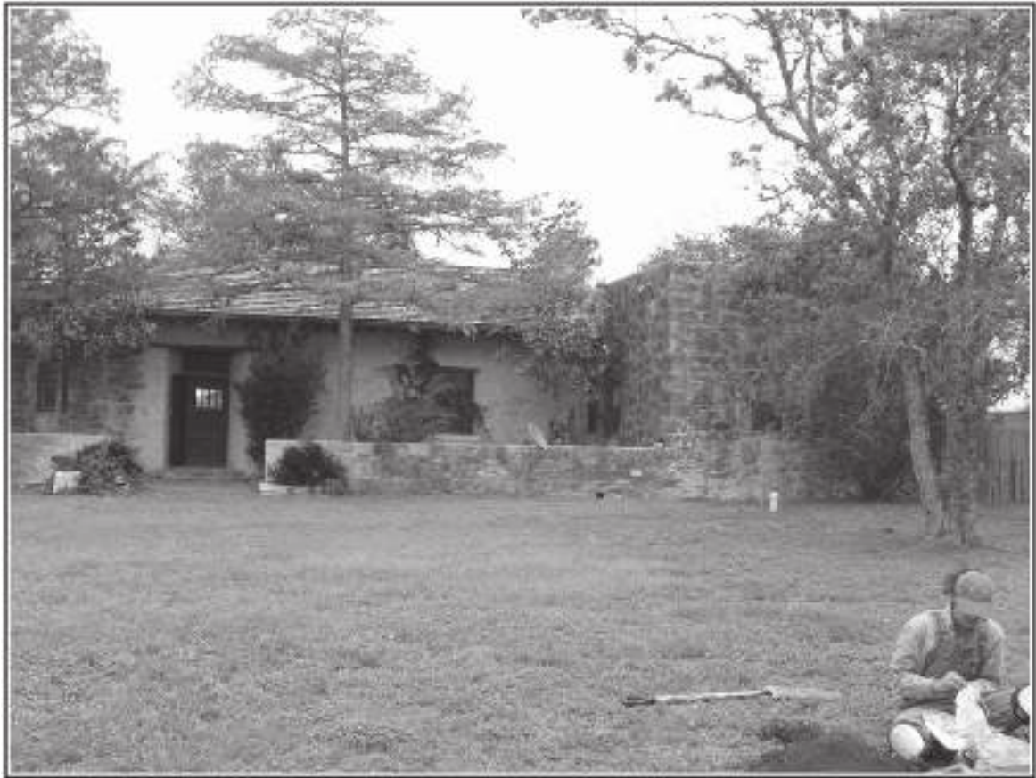
Figure 5-23. Front entrance of the structure constructed by the CCC, 41GD147, facing east (see Figure 5-22).
