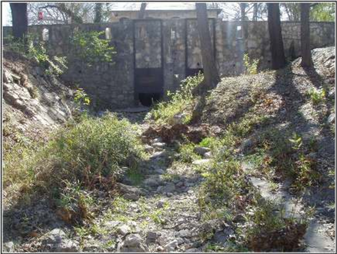
Figure 2-2. San Antonio Water Works Company pump house in present state.
