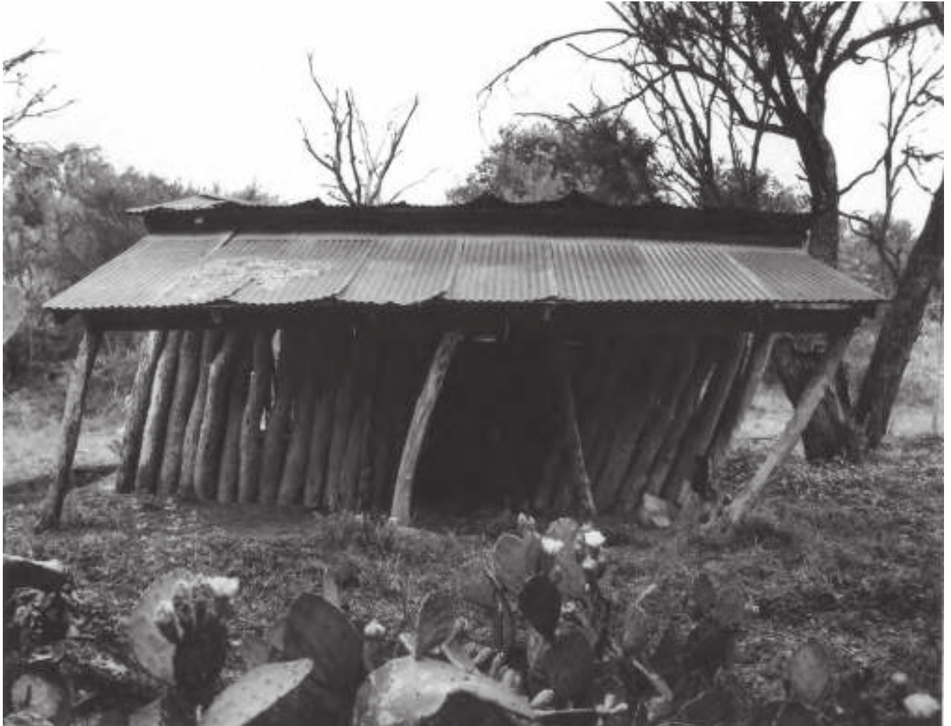
Figure C-6. View of jacal showing front porch, looking north (TX-3539-A-4).
