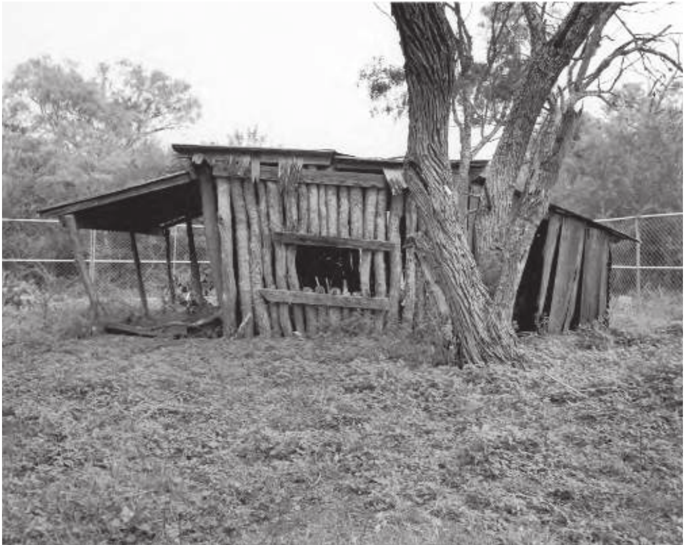
Figure C-4. View of jacal, looking west (TX-3539-A-2).
