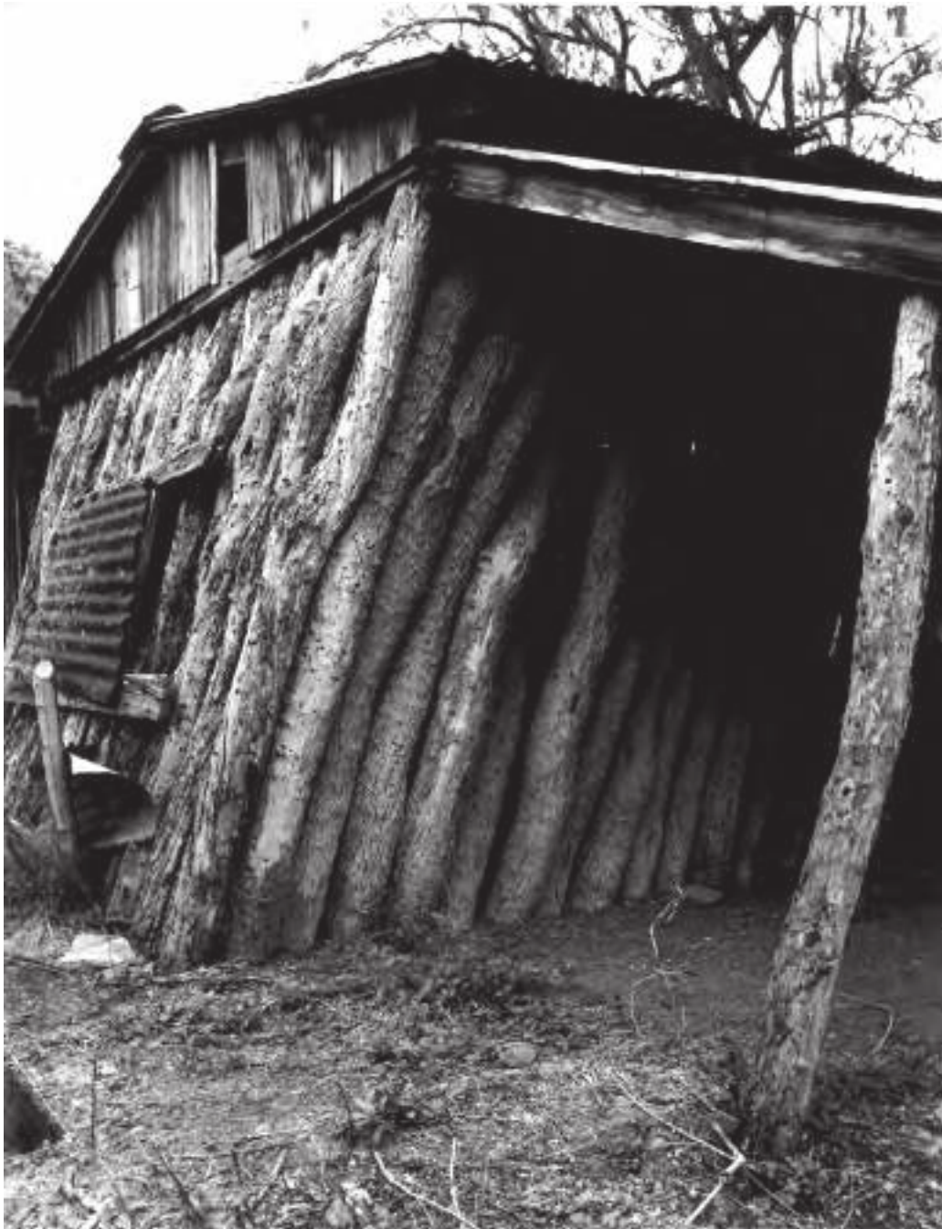
Figure C-11. View of jacal showing detail of overall tilt at southwest corner, looking northeast (TX-3539-A-9).
