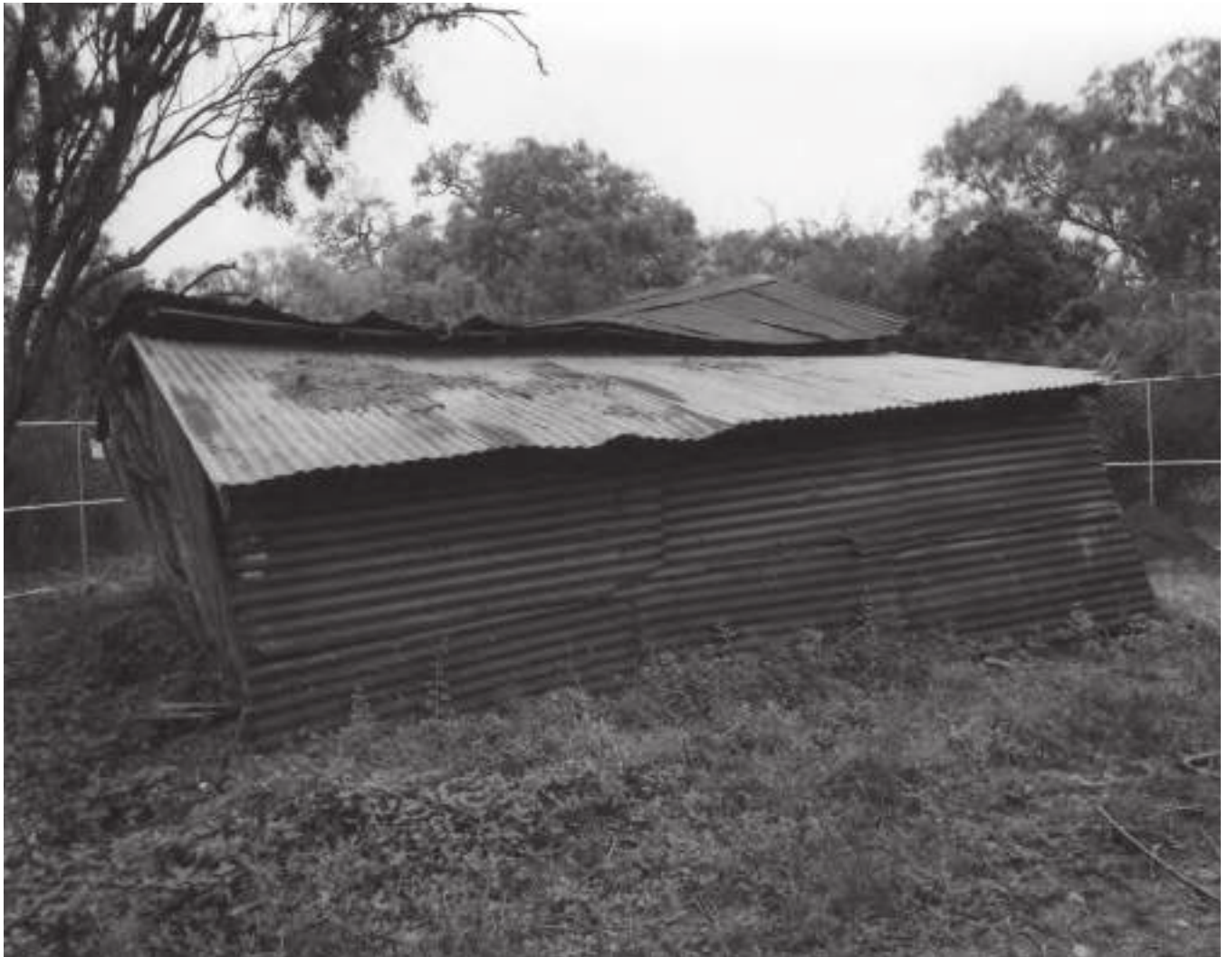
Figure C-8. View of jacal showing rear construction materials and roof, looking south (TX-3539-A-6).
