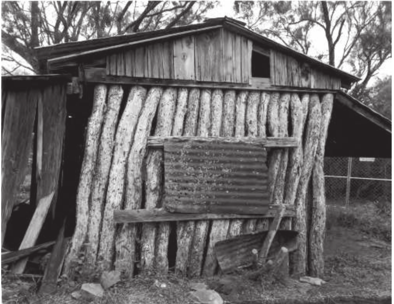
Figure C-10. View of jacal window and gable detail with modern and historic construction material, looking east (TX-3539-A-8).
