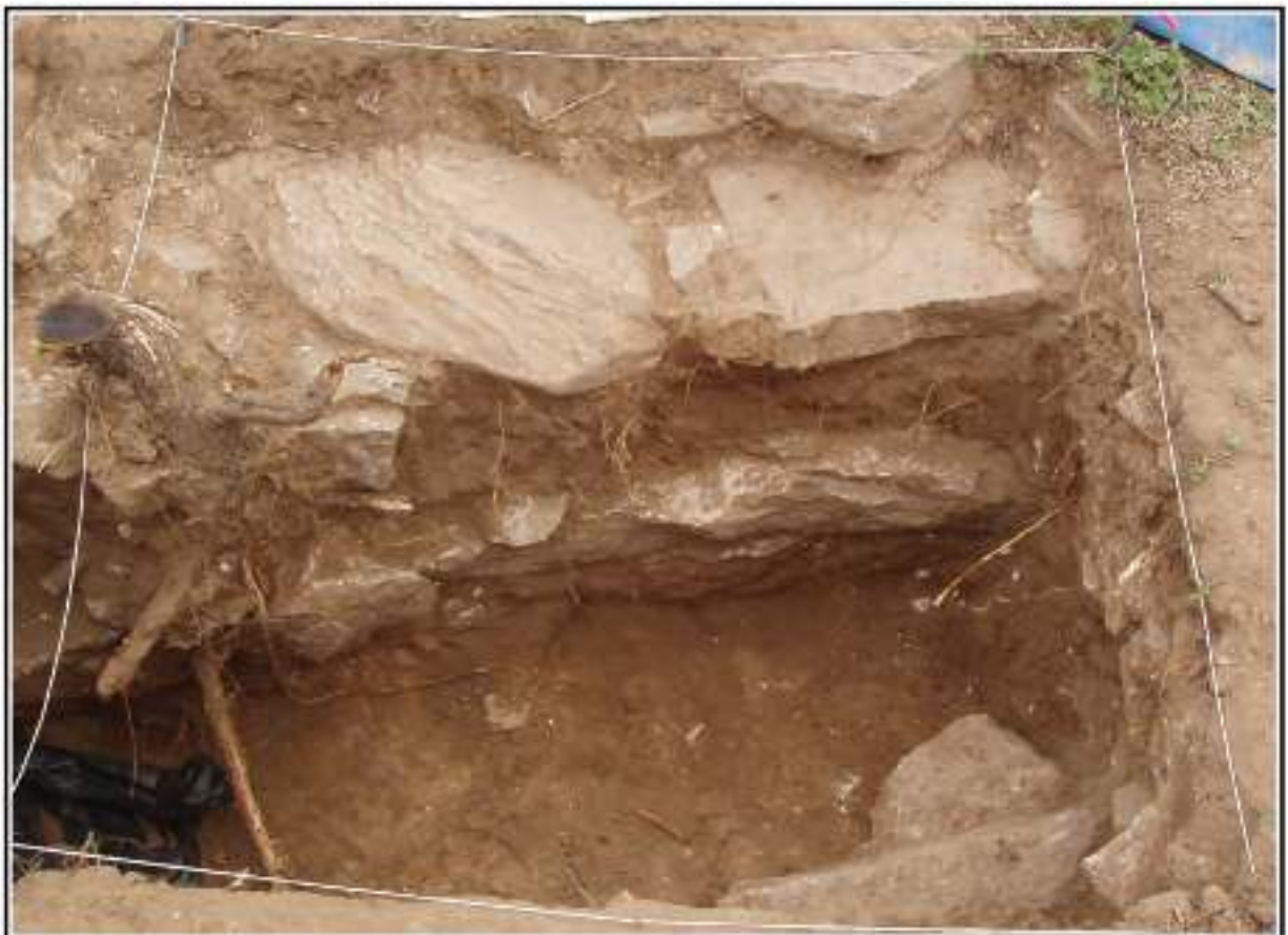
Figure 5-12. Foundation exposed in the east wall of Unit 64.
