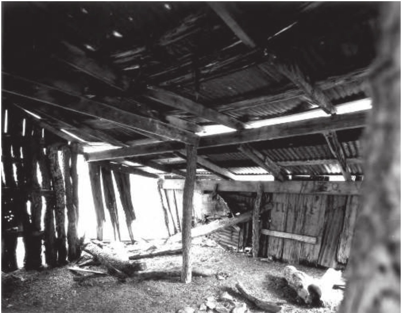
Figure C-12. Interior view of jacal looking northwest to rear (TX-3539-A-12).
