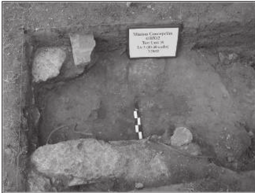
Figure 5-29. Remnant of concrete foundation of restroom facility in Test Unit 39.
