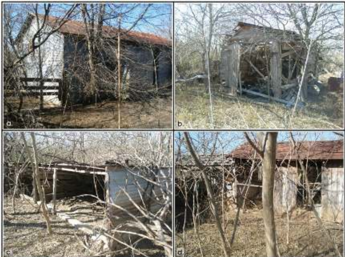
Figure 4-15. Outbuildings at 41BX1795: a) barn b) shed and c-d) pens.
