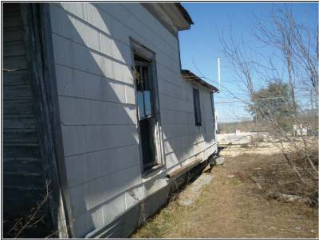
Figure 4-11. The north eastern portion of the structure.
