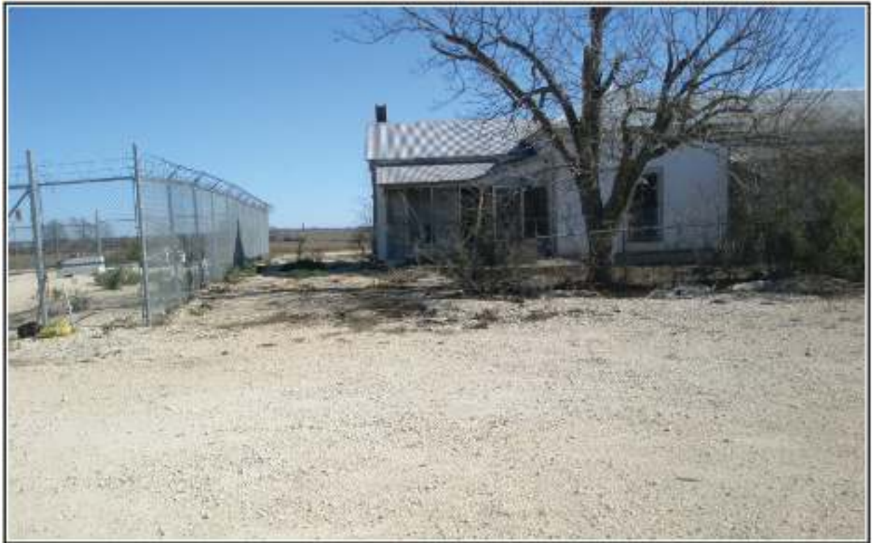
Figure 4-7. The east façade of the main structure at 41BX1794 and fenced construction area (on left).
