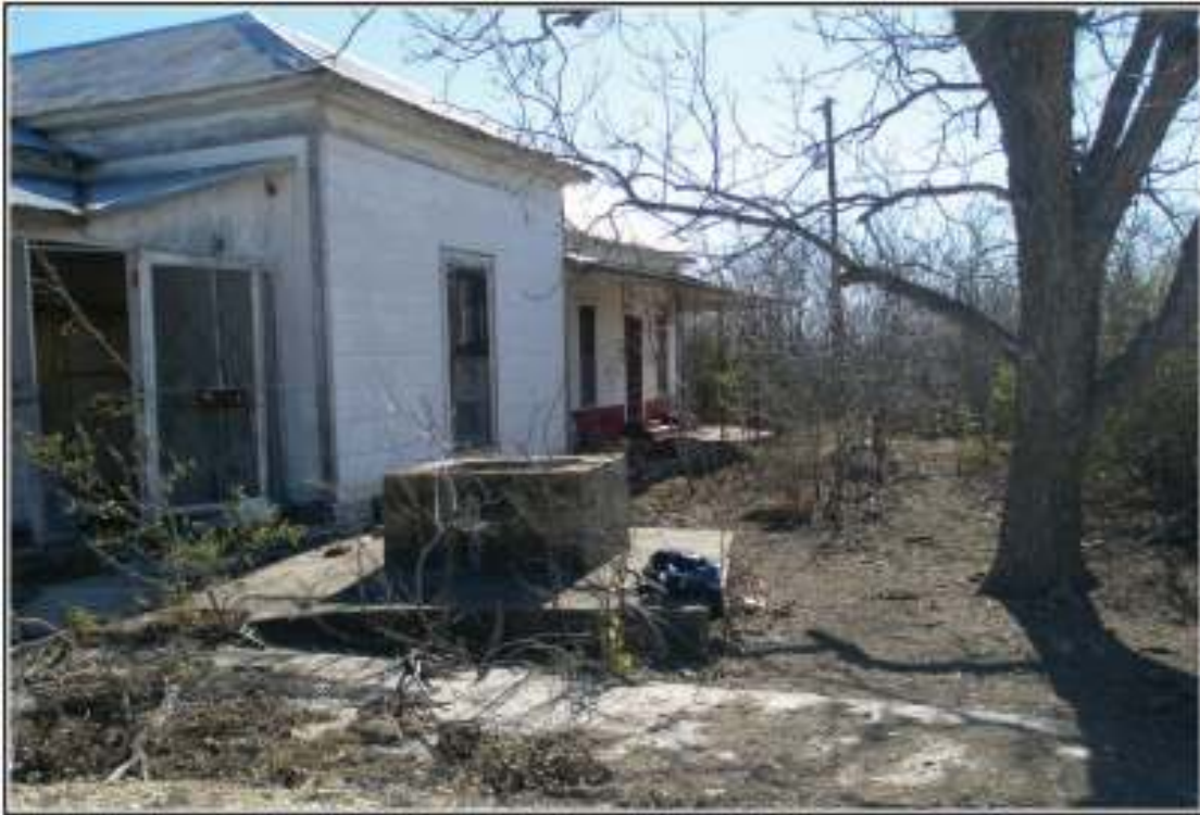
Figure 4-9. The western façade of the structure.
