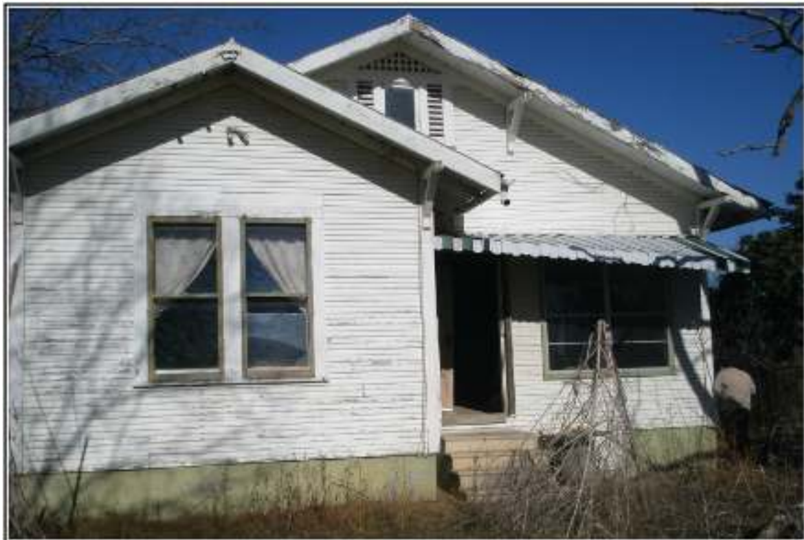
Figure 4-13. The south façade of the main structure at 41BX1795.
