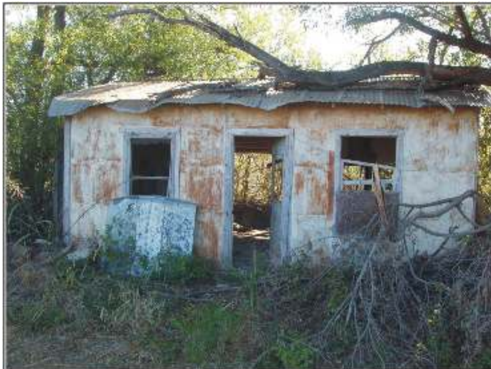
Figure 5-6. Two room structure at 41BX1789 (facing east).
