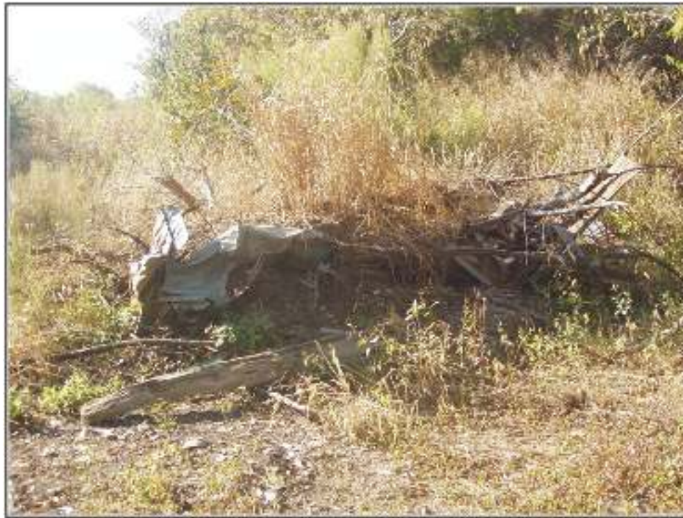
Figure 5-9. Debris pile south of structure containing wooden beams, glass, metal and ceramics.
