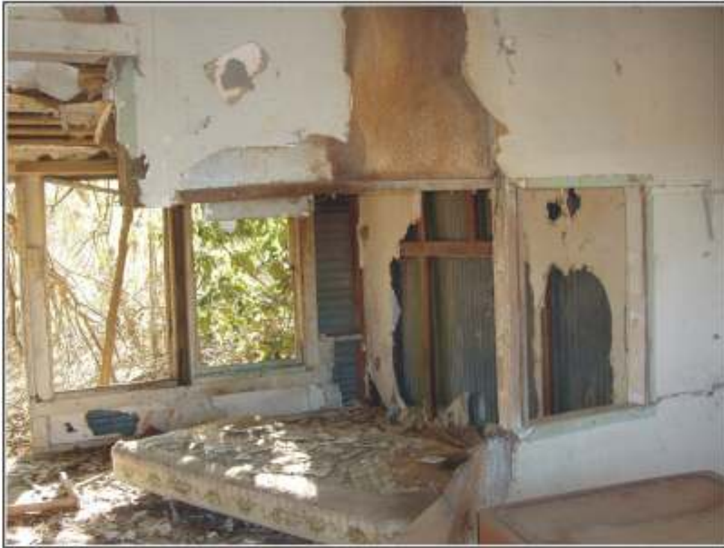
Figure 5-7. East room of structure at 41BX1789, note exposed metal walls and wooden frame (facing southeast).
