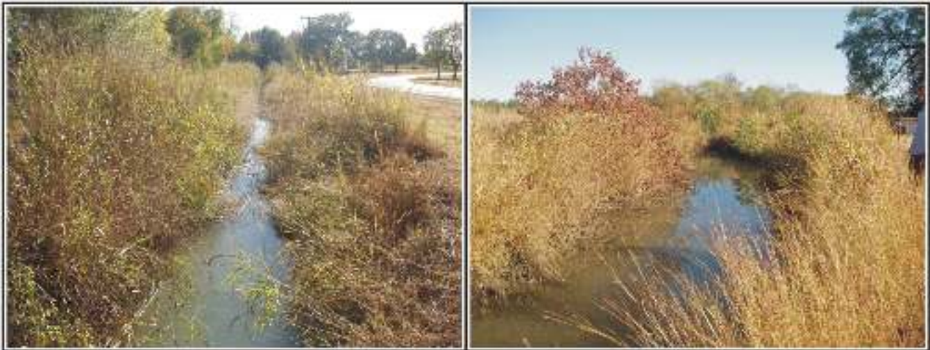
Figure 1-2. Canal that runs along the northern and western boundary of the project area.
