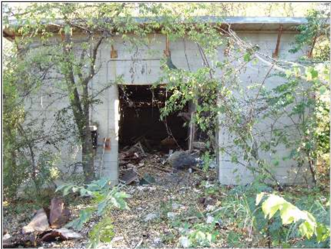
Figure 3-14. Entrance to Structure 12.
