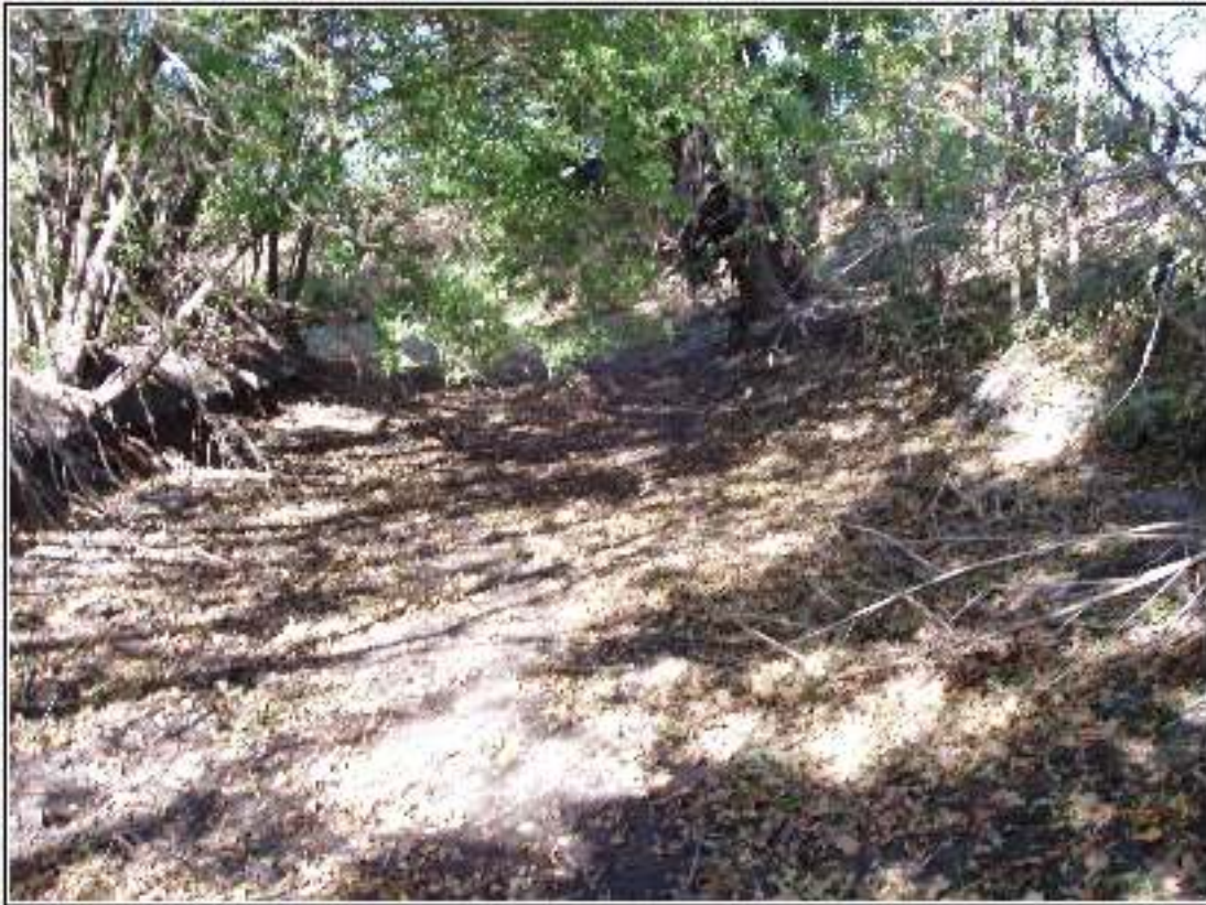
Figure 3-2. The remnants of the Acequia Madre de Valero, showing the active erosion taking place in the ditch as of November 2008.
