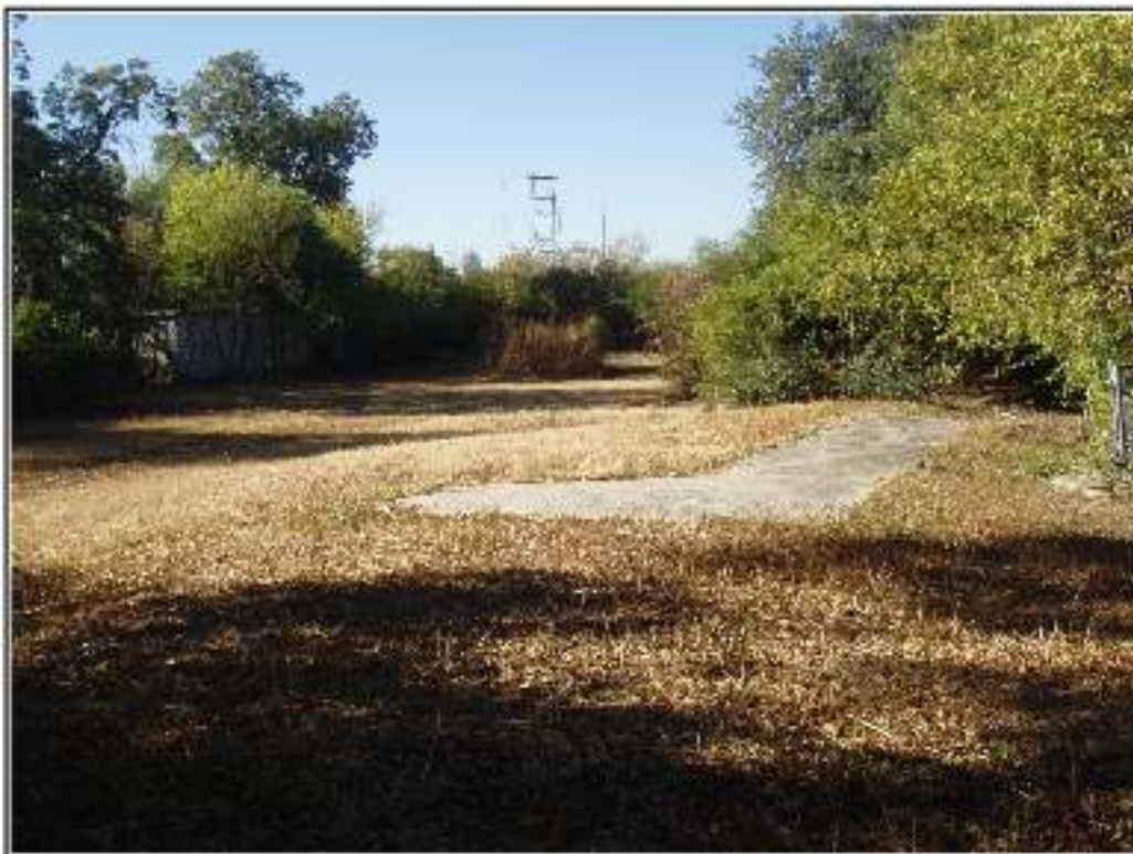
Figure 3-12. The eastern end of Structure 7, a sidewalk leading to the entrance to the roller coaster. Note the area to the left of the photograph, where the roller coaster once stood. Also note the remains of the old TV tower (Structure 13) at the center back of the photograph.
