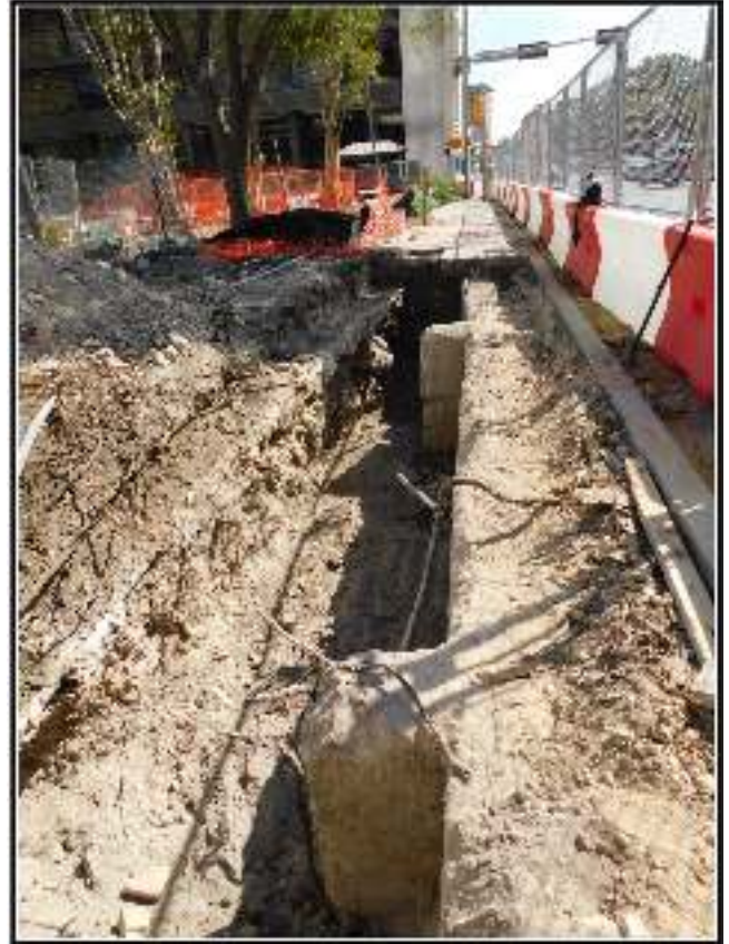
Figure 4-2. Electrical line project area along the east side of N. Flores Street. Note concrete pier and beam footings for the Majestic theatre, site 41BX2347 (view south).
