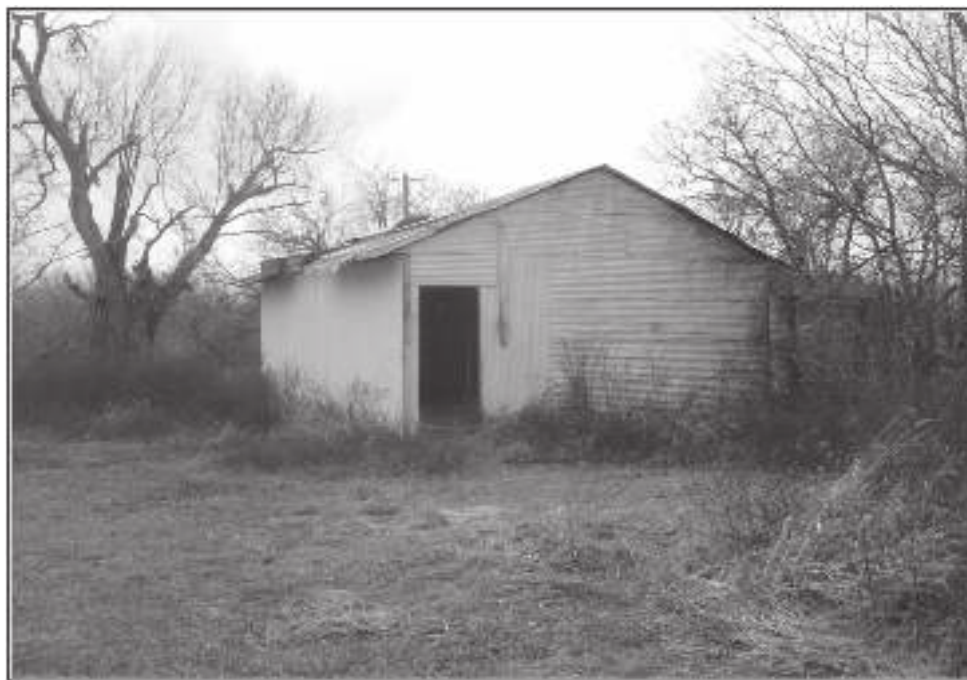
Figure 4-18. Two car garage (Outbuilding 7) on 41BX538.
