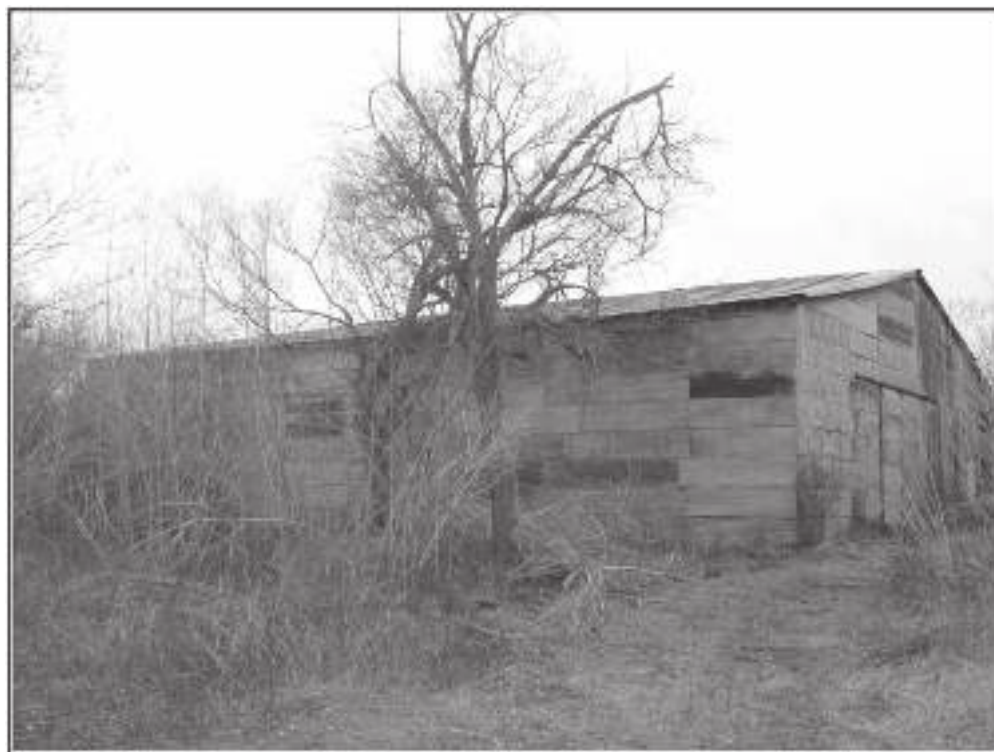
Figure 4-14. Metal barn (Outbuilding 3) on 41BX538.
