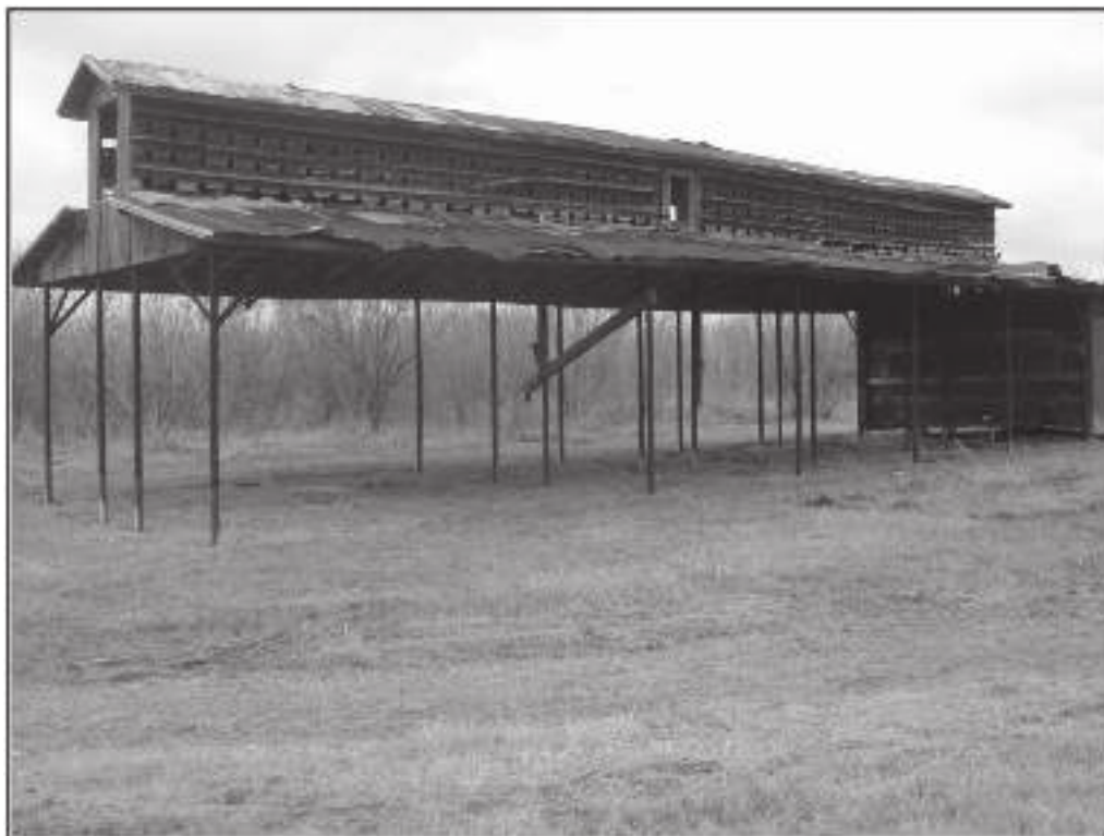
Figure 4-12. Pigeon coop 1 (Outbuilding 1) moved from 41BX681 to 41BX538.
