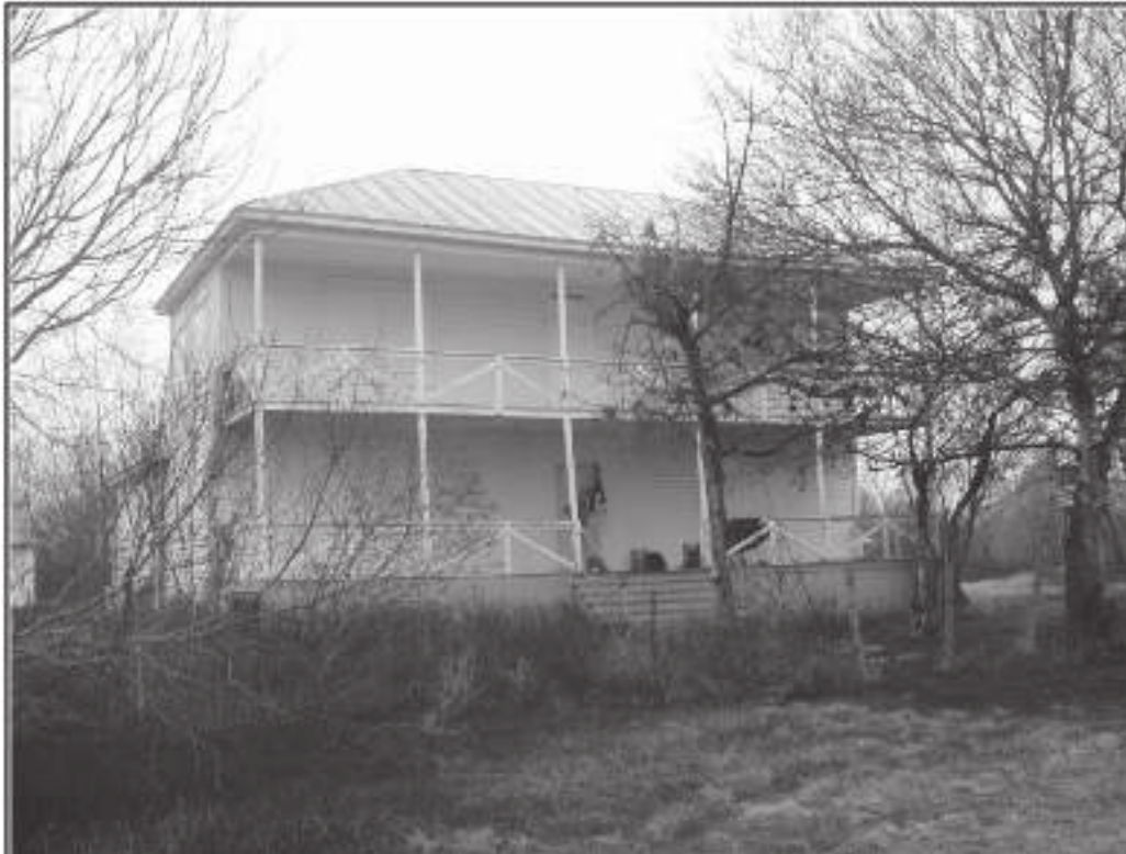
Figure 4-11. Main structure at 41BX538.
