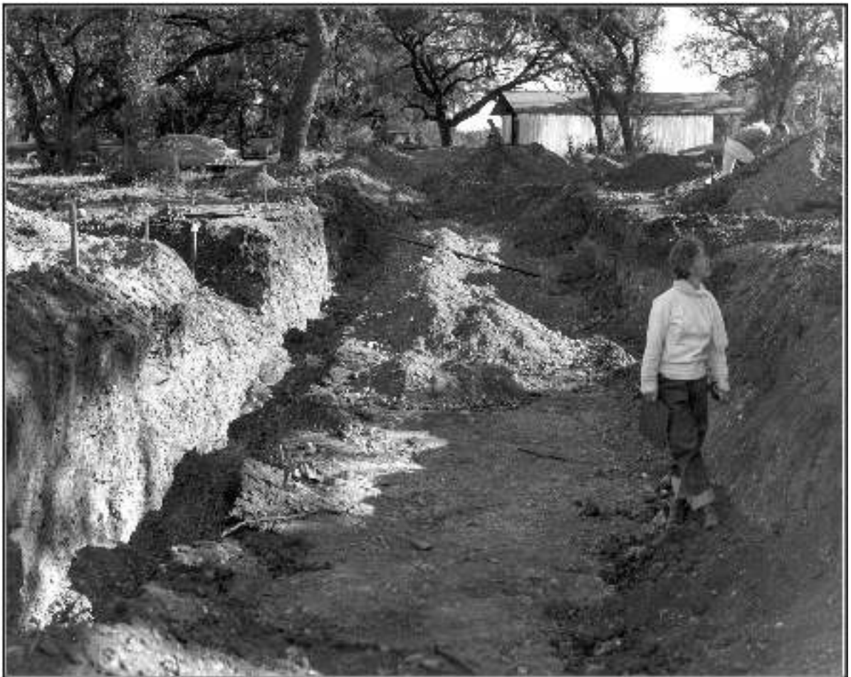
Figure 4-4. Open trench at Granberg I, 1962.
