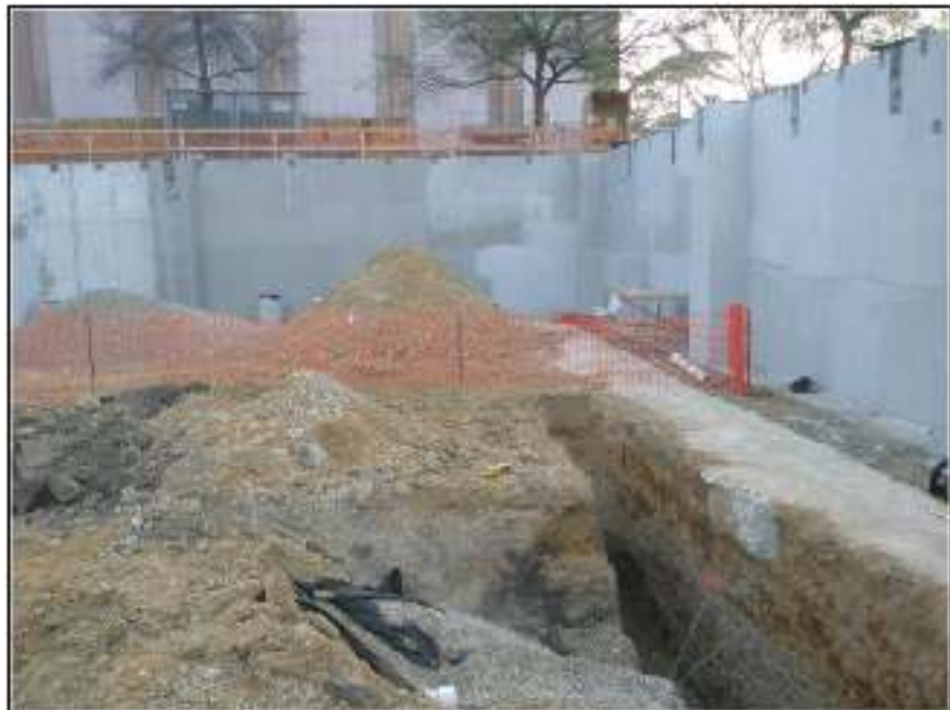
Figure 4-22. Feature 10 encountered during sump pit excavations.
