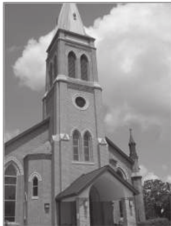
Figure 3-10. Photograph of St. James Catholic Church.
