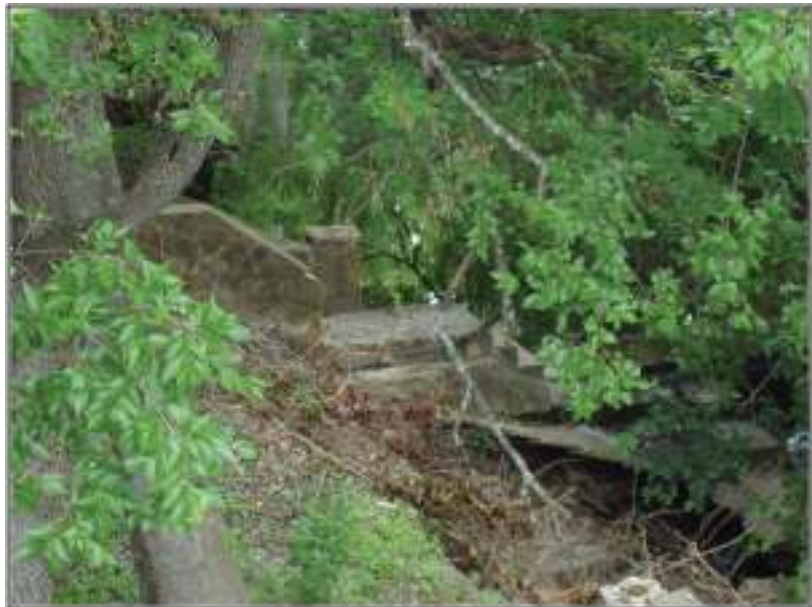
Figure 3-24. Current photograph of Walnut Branch showing remains of stairs leading to the creek.
