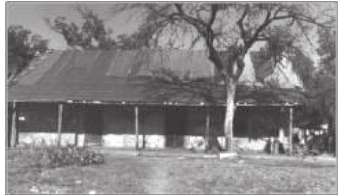
Figure 3-6. Photograph of the front of the Ranger Station.
