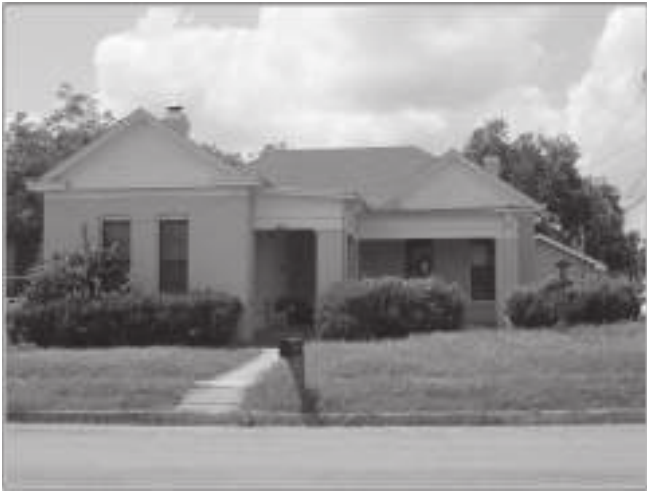
Figure 3-14. Photograph of 413 West Nolte Street.
