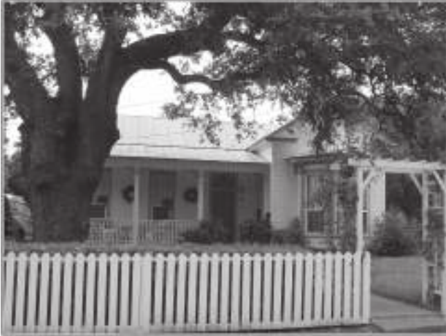
Figure 3-8. Photograph of 323 West Nolte Street.
