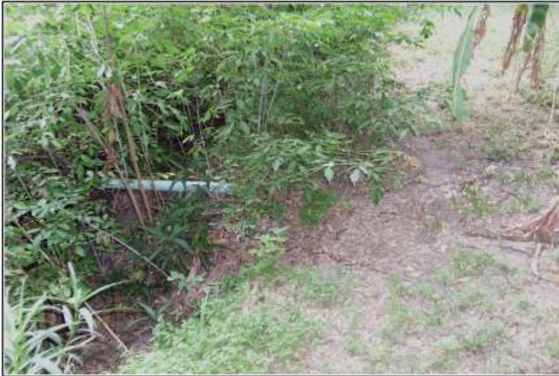
Figure 5-15. PVC drainage pipe beneath site 41GU115.
