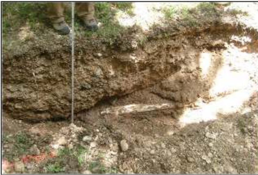
Figure 5-9. Photograph of buried PVC drainage pipes.
