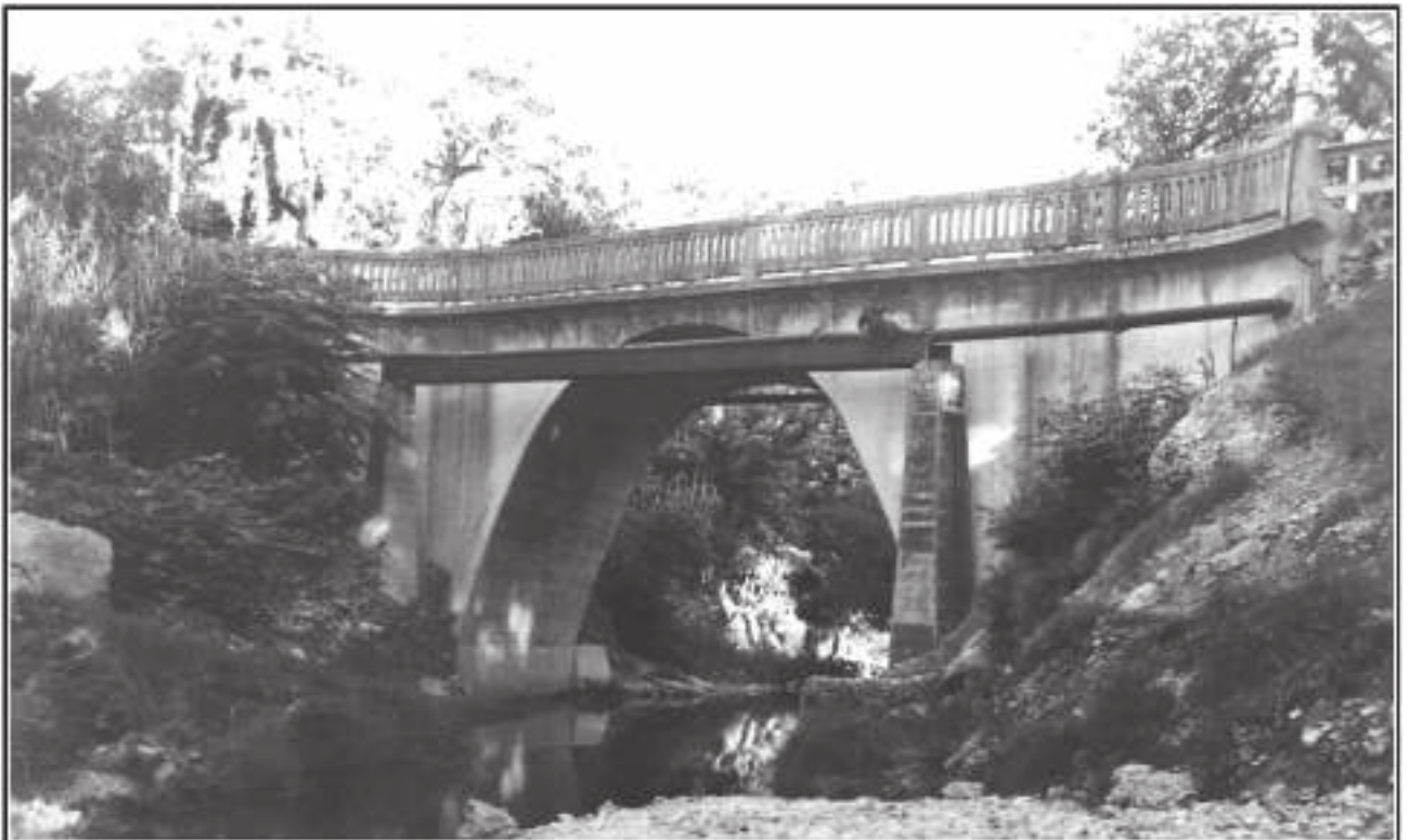
Figure 3-22. Photograph of the Nolte Street Bridge ca. 1935.
