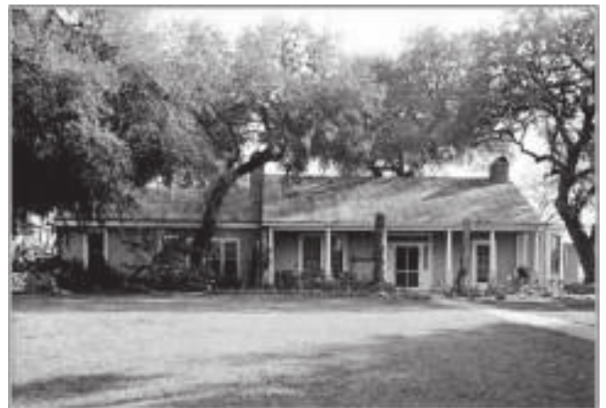
Figure 3-19. Photograph of the Smith-Hollomon House ca. 1936 (HABS TEX, 94-SEGUI, 4-1).
