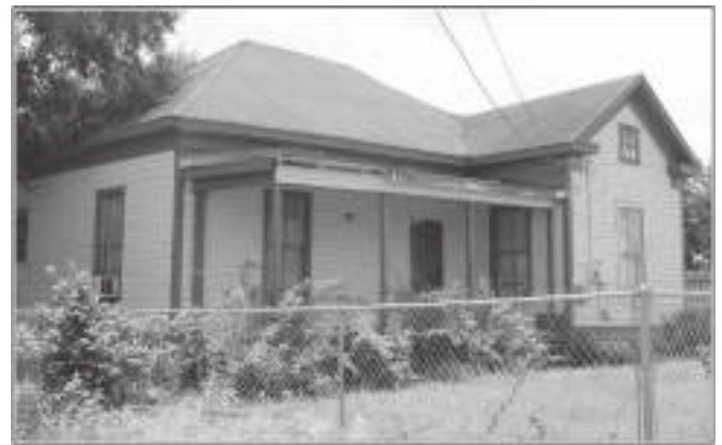
Figure 3-7. Photograph of 203 South Guadalupe.
