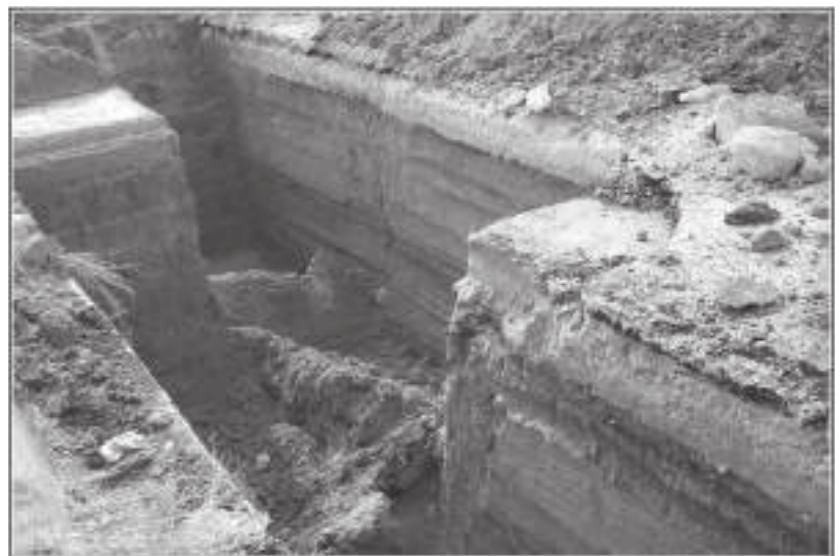
Figure 5-13. Photograph showing Trench B at approximately 34+080, as the first half of a new section has been completed, showing the wall at the center of the trench (foreground) and the wall at the western edge of the trench (background). Looking southwest.
