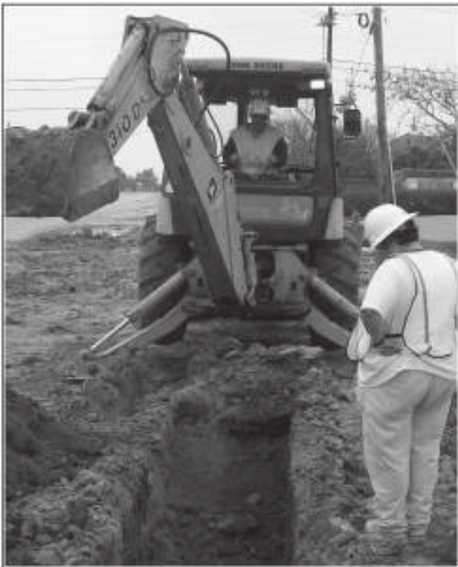
Figure 4-2. Monitoring trench excavation near the location where it is believed Jackson’s 1933 excavations took place. Facing east.
