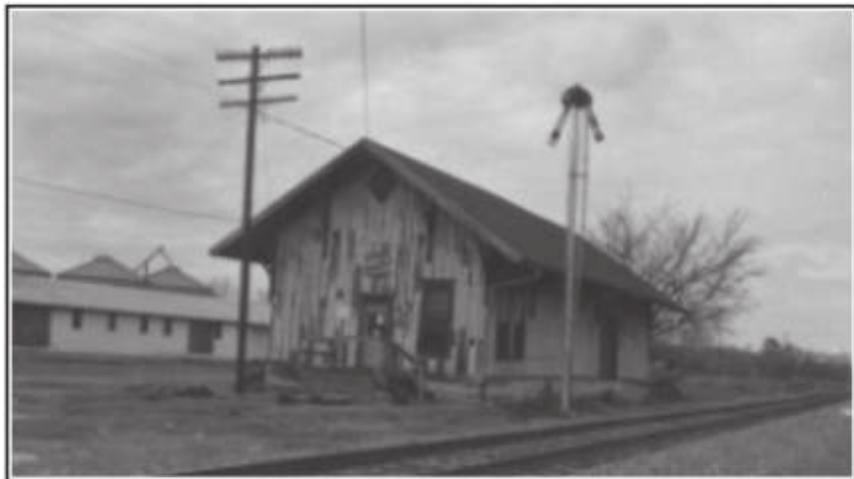
Figure 3-8. Old photograph of M.K.T. Depot with still standing landmarks in background.
