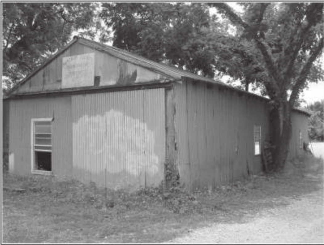
Figure 6-18. Commercial structure at 1317 Farm Road.
