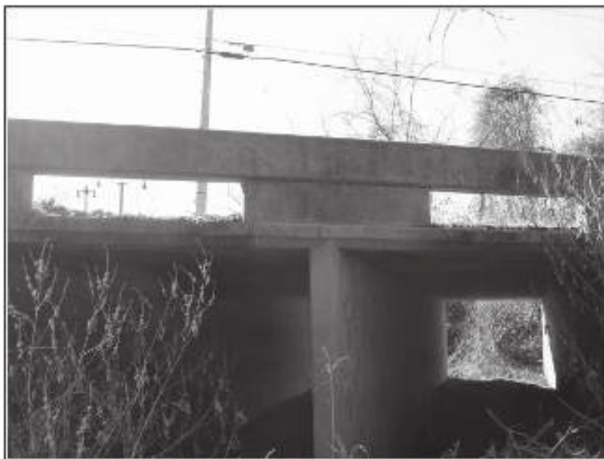
Figure 3-3. Current bridge over Gills Branch.
