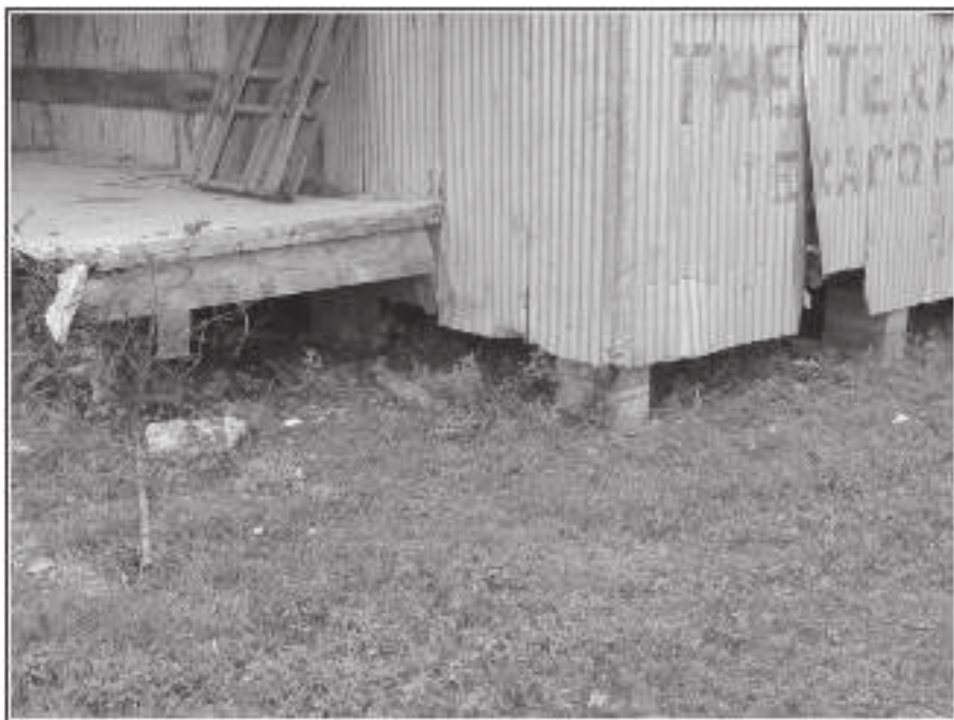
Figure 6-9. Foundation network of cinderblocks and beams under “Texas Company” structure.
