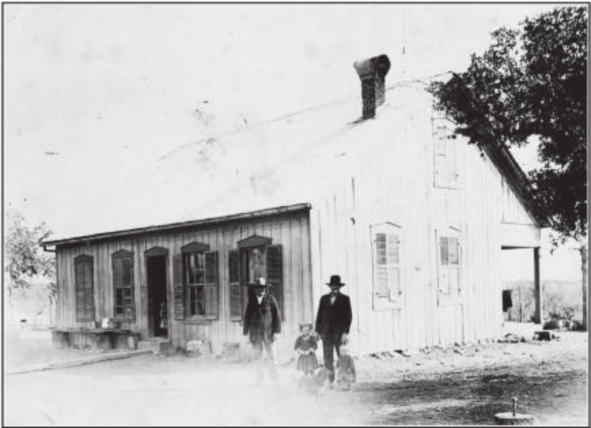
Figure 2-2. Photograph of the Heirholzer-Kruse farmhouse.
