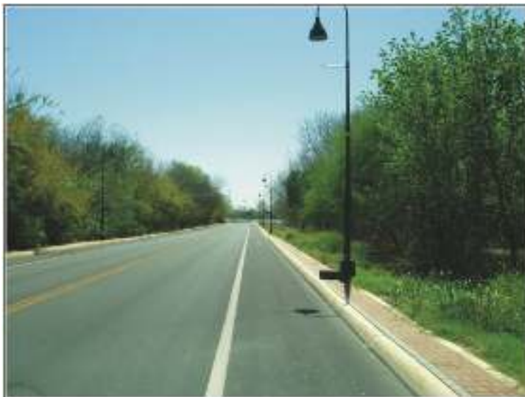
Figure 5-1. The new hike and bike trail along Padre Road.
