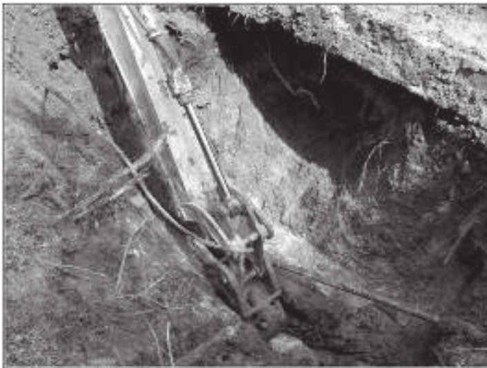
Figure 4-18. Backhoe digging below Mission Road, showing degree of previous disturbance in trench.
