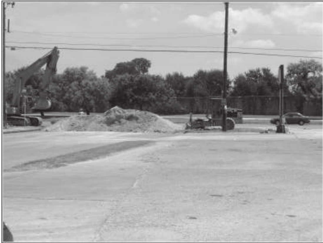
Figure 4-17. Monitoring utility placement on Roosevelt Avenue, looking northeast, with west wall of Mission San José in background.
