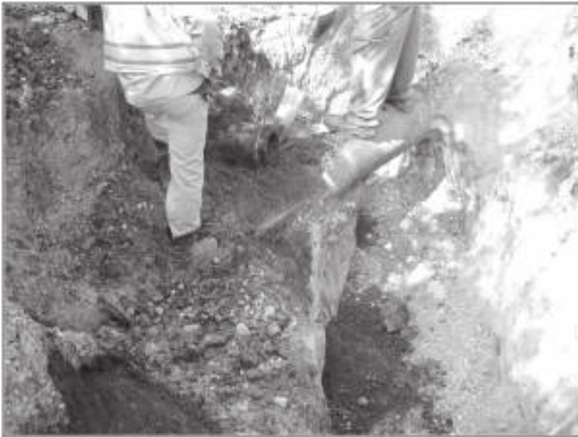
Figure 4-19. Working around old utility lines in a trench on Mission Road near E. White Avenue.
