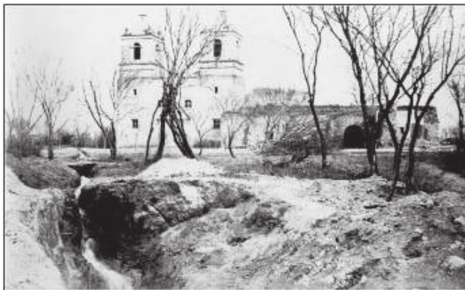
Figure 2-3. Photograph of Mission Concepción probably taken in the late nineteenth century, showing a new acequia crossing the old mission compound.
