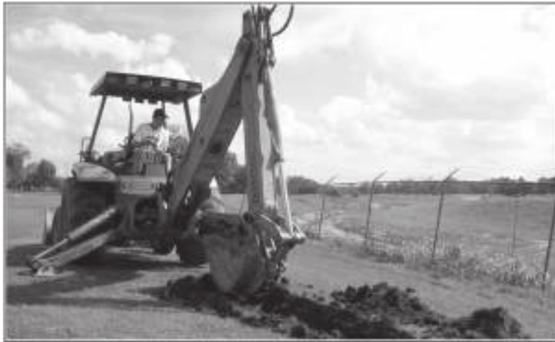
Figure 4-24. Digging Trench C on the north bank of the San Antonio River, near the Mission Road Bridge. Looking southeast.
