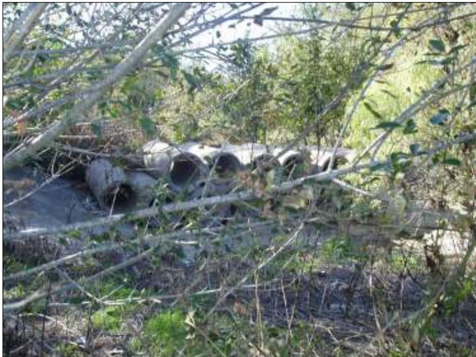
Figure 18. Culverts were stacked to allow floodwaters to drain while also serving to keep horses out of the creek, according to a former horse caretaker on the property.
