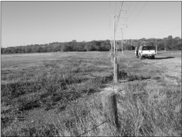
Figure 11. The eastern edge of the lot east of Zarzamora Creek south of Callaghan is paved and the entire lot is littered with construction debris.
