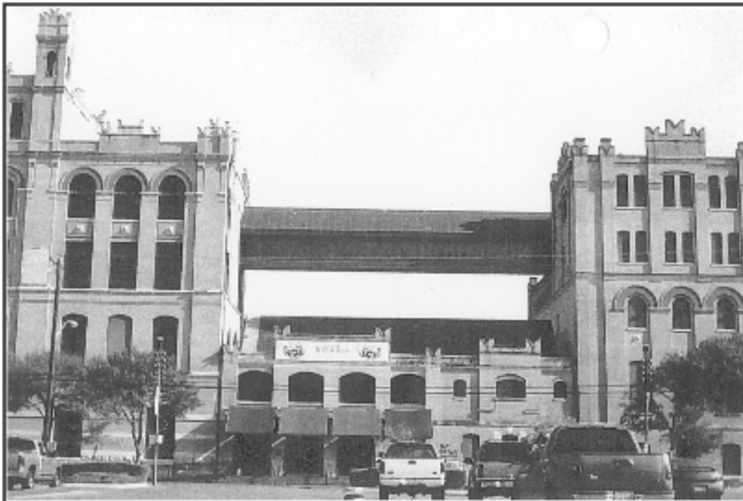
Figure 2-10. Lone Star Brewing Company (Historic Resource #22, southwest façade).
