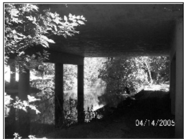
Figure 4-2. West bank of San Antonio River under the Newell Street Bridge.
