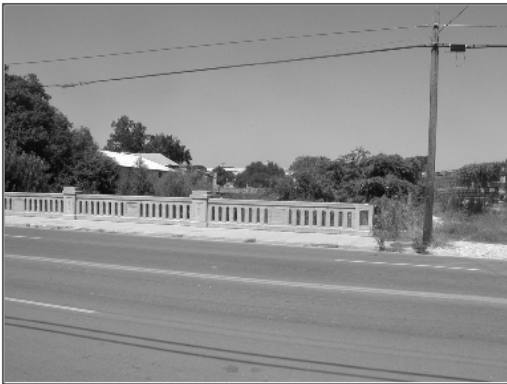
Figure 2-4. The Grayson Street Bridge located on Grayson Street (Historic Resource #43).
