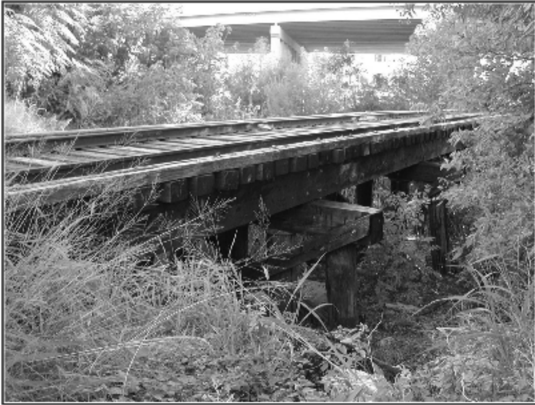
Figure 2-8. Wooden trestle bridge located between Camden Street and IH-35.
