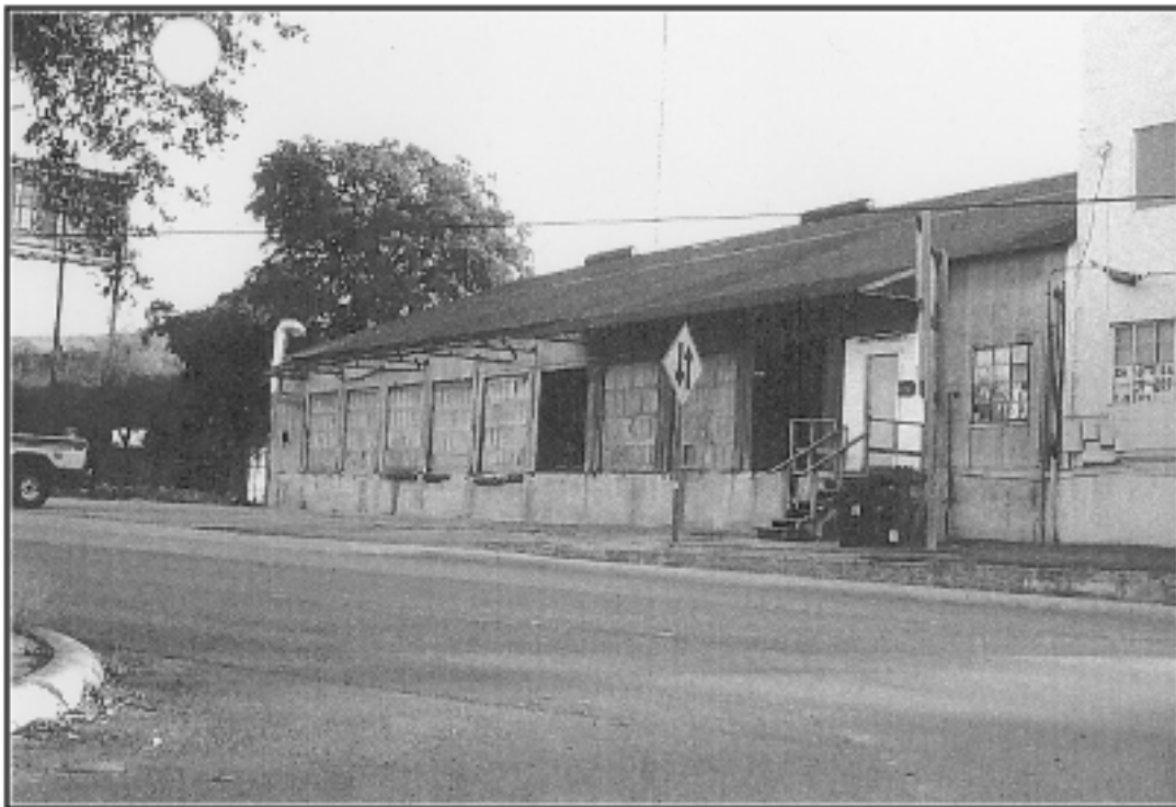
Figure 2-24. Historic Resource #32 located on East Quincy Street (north façade).
