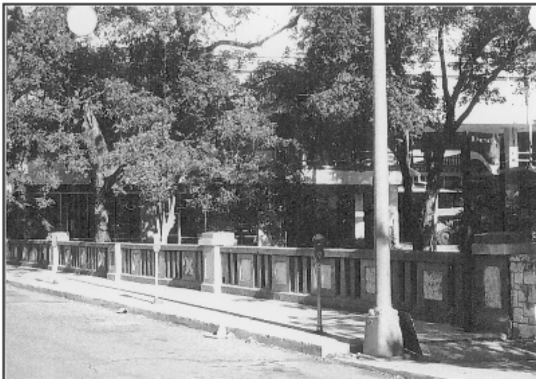
Figure 2-2. The Fourth Street Bridge located on Lexington Avenue (Historic Resource #1).
