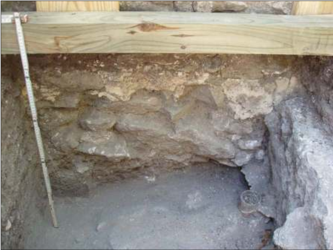
Figure 12. Photograph of the foundation.
