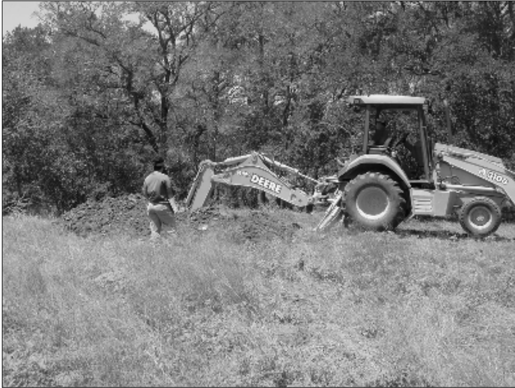
Figure 5-2. Backhoe trench excavation at 41BP679.
