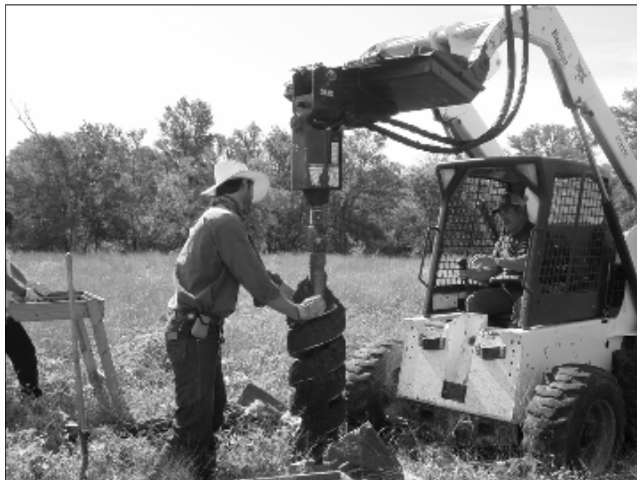
Figure 5-1. Mechanical auger in use on site.
