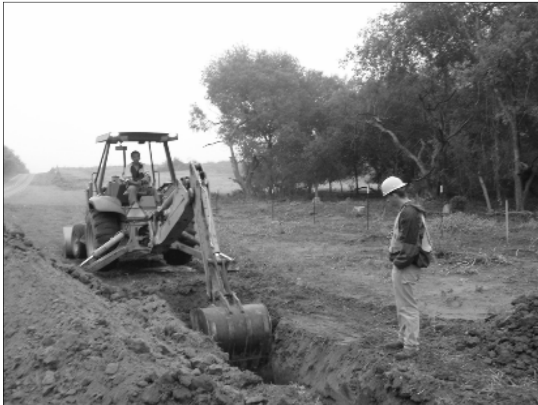
Figure 3-2. Backhoe trenching at FM 536.
