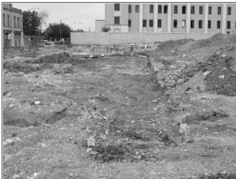
Figure 5-9. Photograph of the initial bladed area, looking north.
