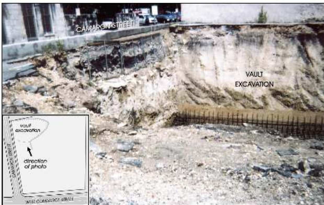
Figure 1-2. Photo of vault excavation area at the time of CAR involvement.
