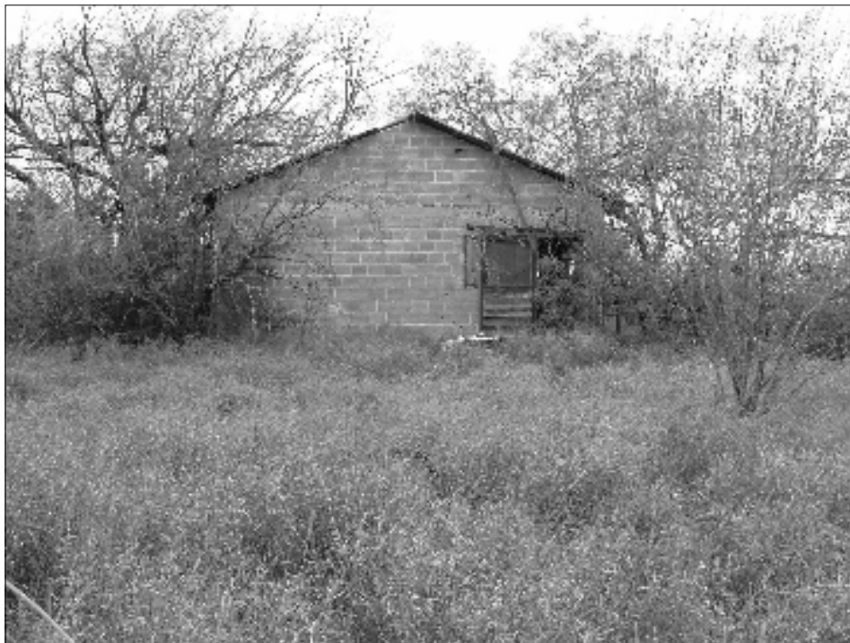
Figure 3-7. Brick structure located south of Field Site 3.
