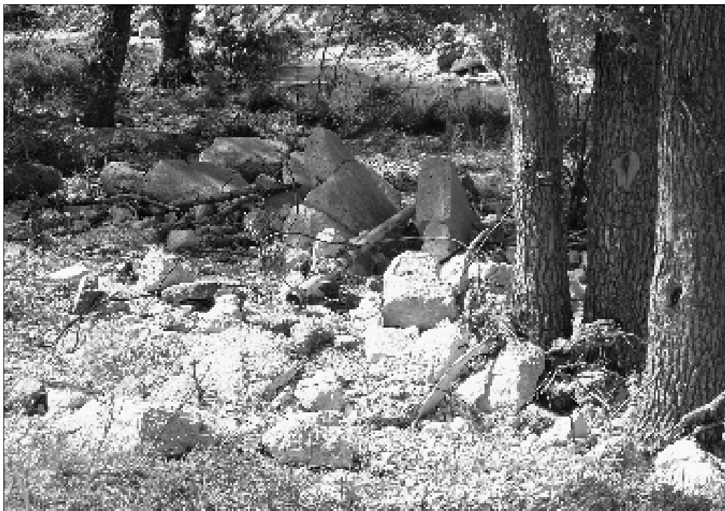
Figure 4-5. Debris on the south bank of Salado Creek in Tract 2.
