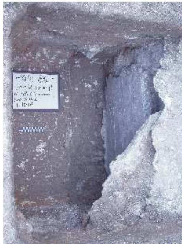
Figure 3-2. Plan view photo of Test Unit 2, showing concrete shelf and reinforcement.
