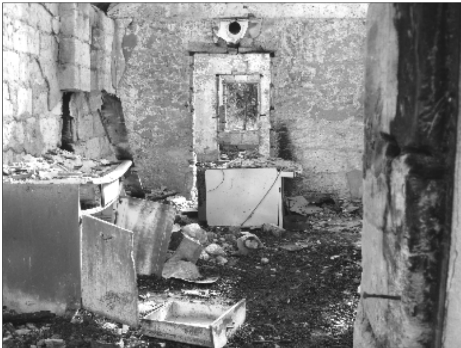
Figure 46. Chimney pipe above door to Addition 3. Note keystones above door in Addition 2 and window in original structure.
