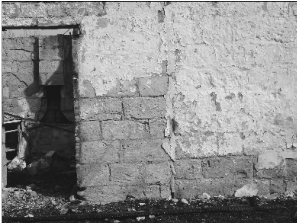
Figure 43. Abutment line and easternmost doorway of Addition 3 to Benke/Naegelin homestead.
