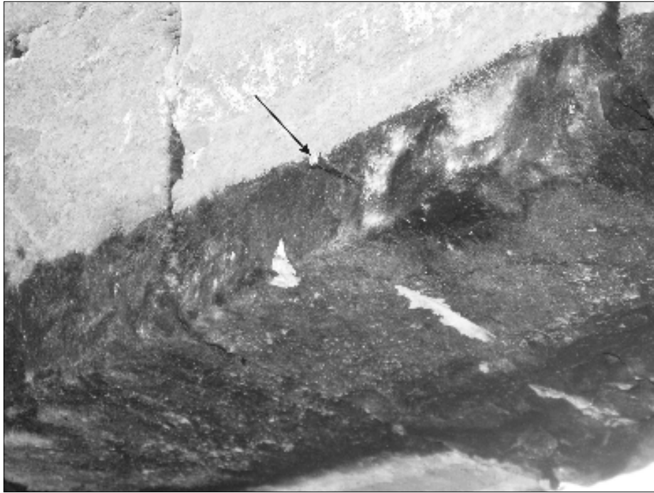
Figure 42. Forged nail that originally supported wood framing around the south window of Addition 1.
