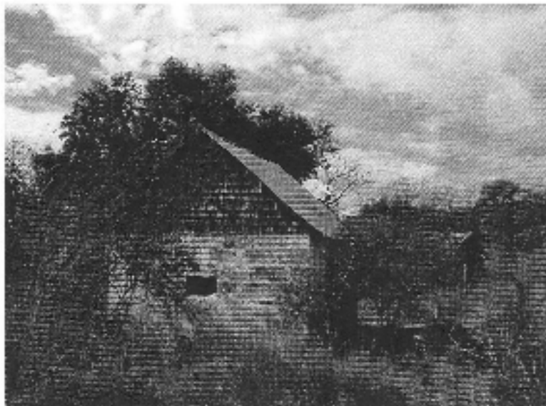
PHOTO 8: View of small structure currently still standing on the site.
