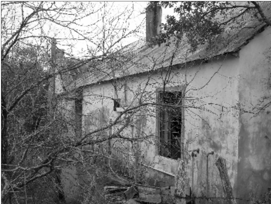
Figure 17. Northern façade of residence (Resource 1).
