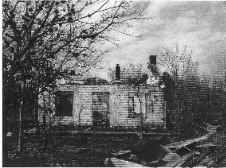
PHOTO 7: Additional view of structure after the fire.
