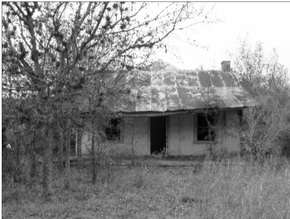
Figure 15. Eastern façade of the stone residence (Resource 1).
