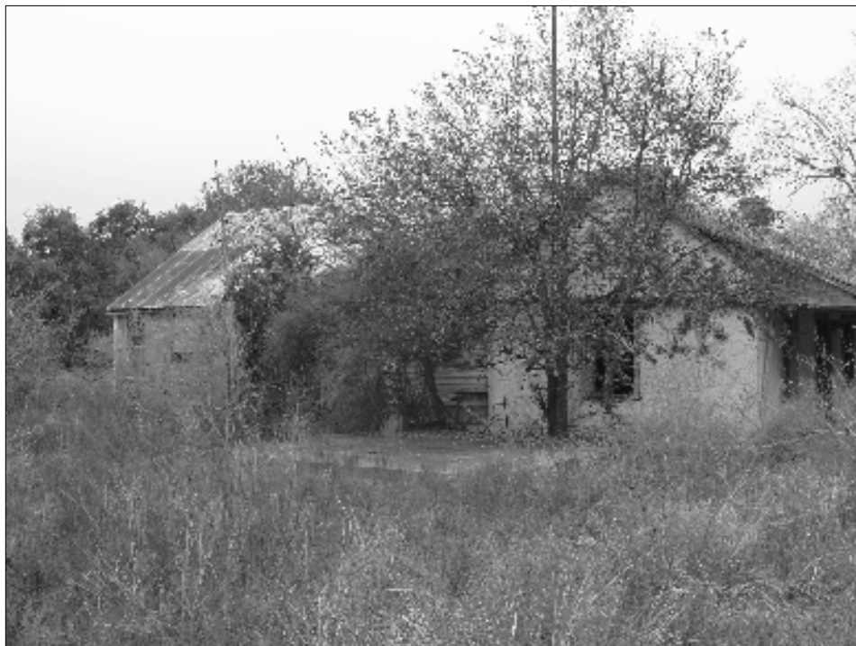
Figure 20. Southern façade of residence (Resource 1).
