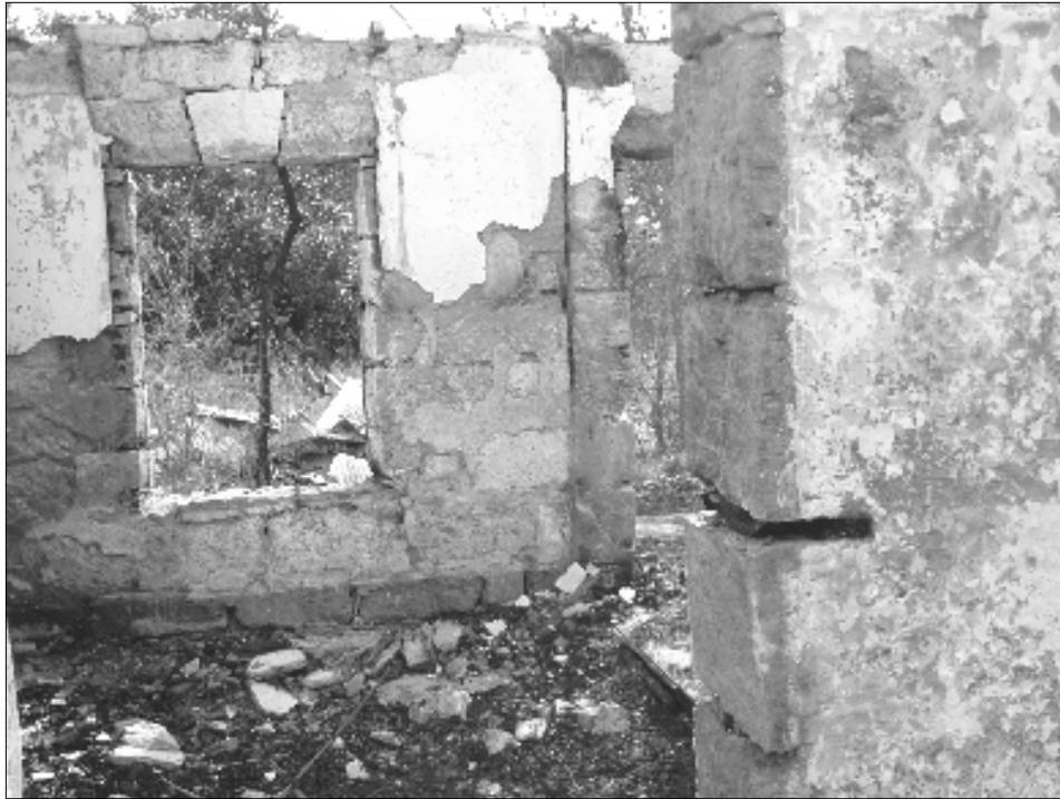
Figure 40. Abutment line and concrete floor of Addition 1 of Benke/Naegelin homestead.
