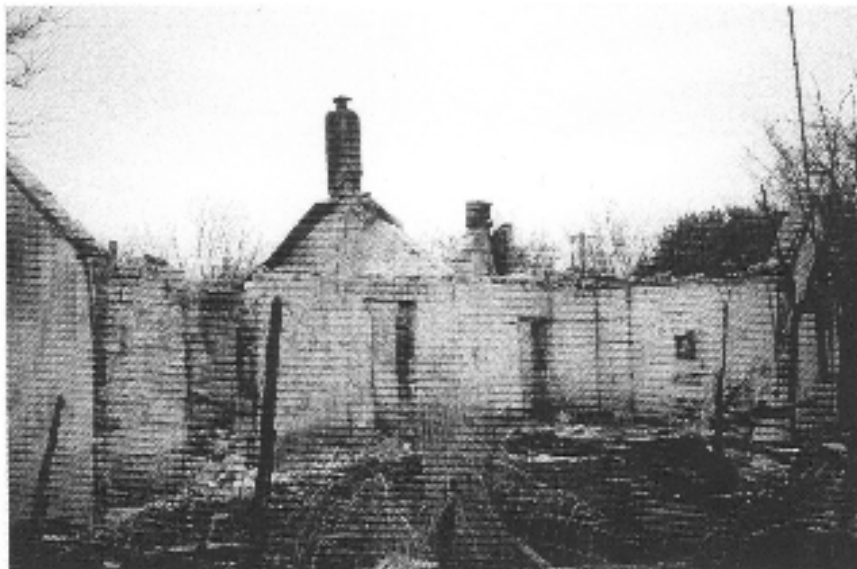
PHOTO 12: View of structure condition up to March 9, 2005.
