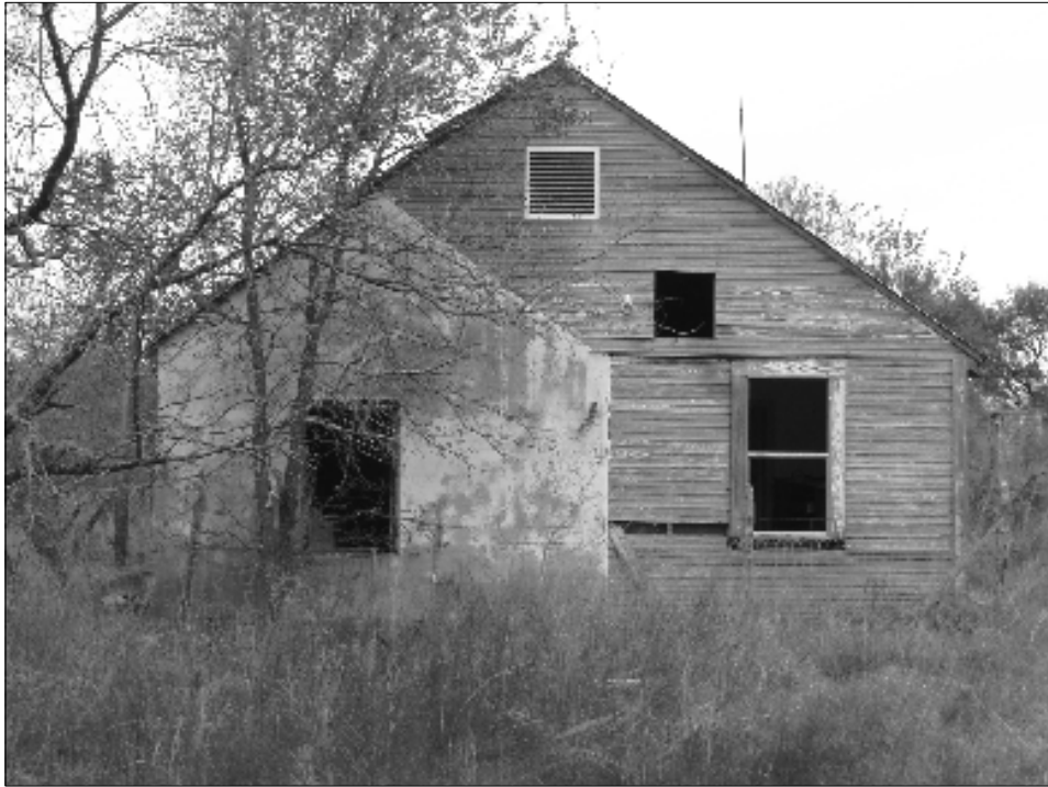
Figure 21. Western façade of residence (Resource 1).
