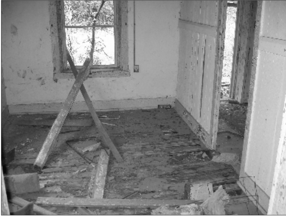
Figure 16. Detail of room division and condition of flooring (Resource 1).
