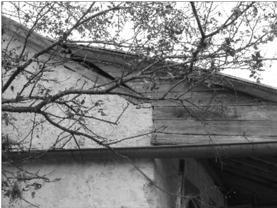
Figure 19. Roof detail of porch addition to the original house.
