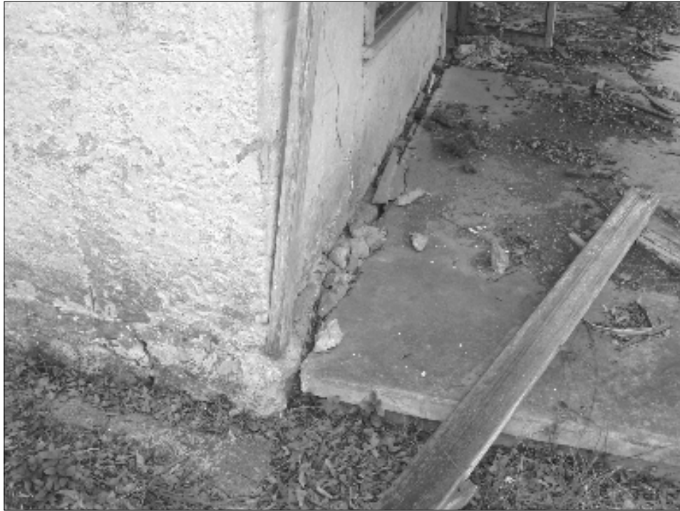
Figure 18. Porch floor and house foundation (Resource 1).
