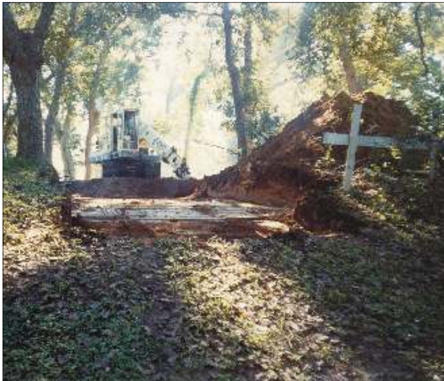
Figure 5-4. Photograph of Gradall scraping in progress.
