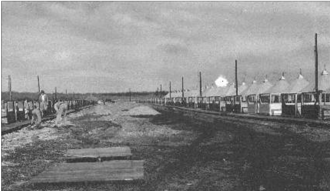
Figure 3-9. Street scene at the prisoner of war camp at Dodds Field, Fort Sam Houston, during construction in 1943. Completed tent pads can be seen on the right. Photo courtesy of Fort Sam Houston Museum.
