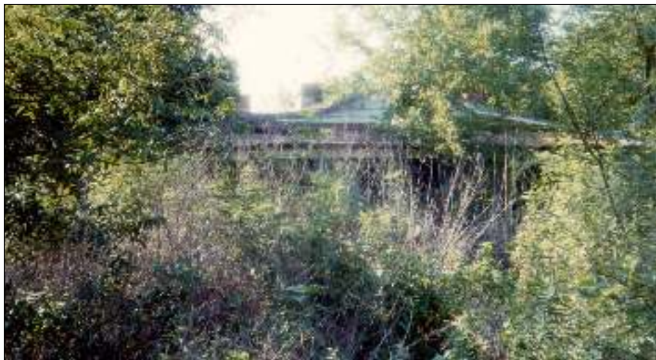
Figure 4-8. 1950s structure on site 41BX347.
