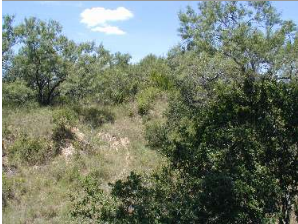
Figure 4-10. Photo of erosion at 41BX348.
