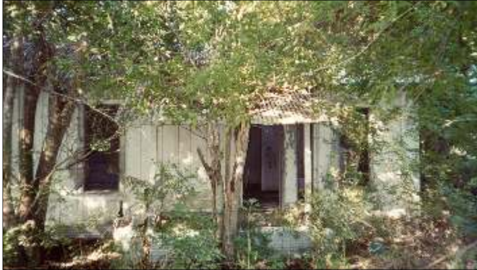
Figure 4-7. 1940s structure on site 41BX347.
