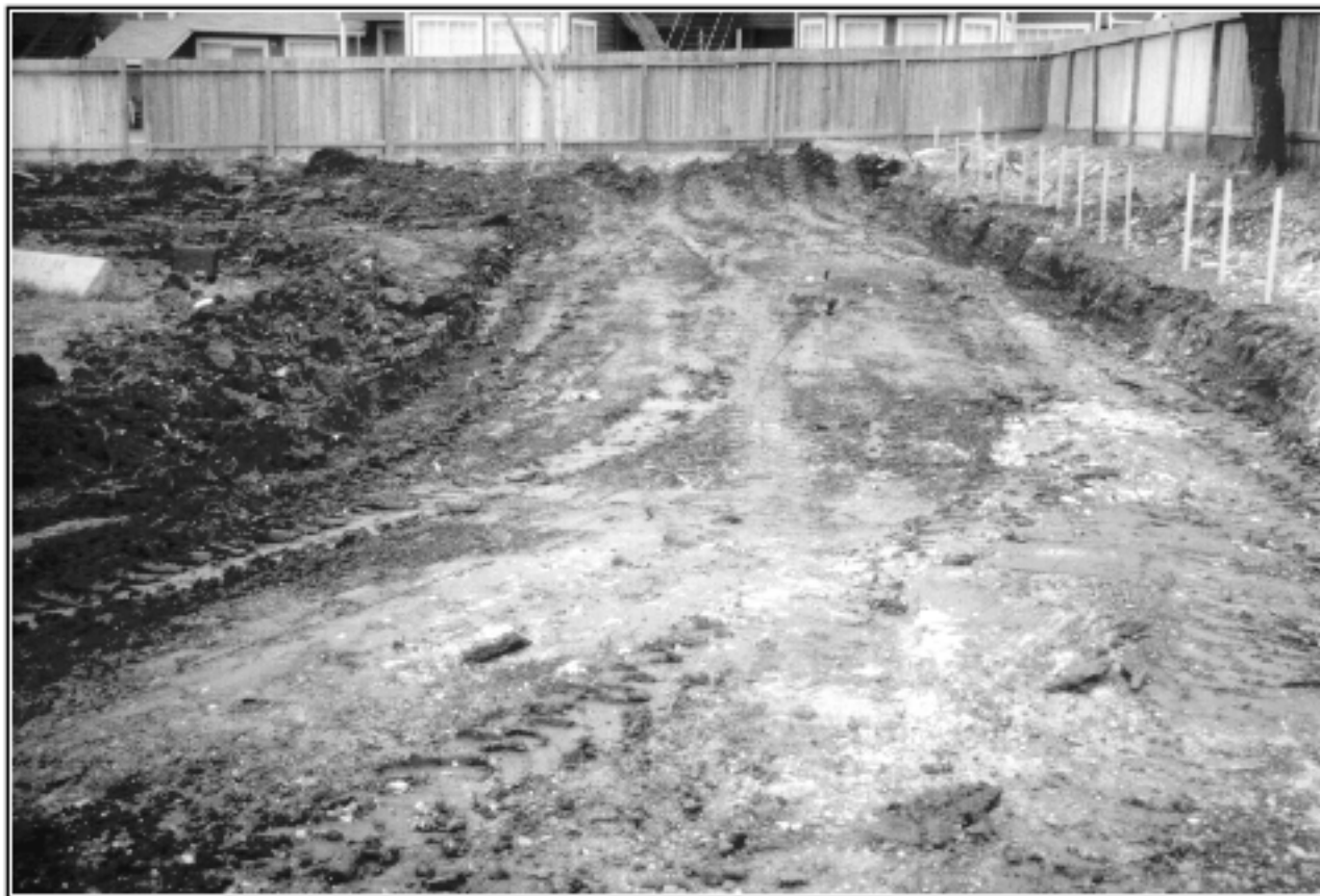
Figure 6. Area of machine scrape looking west.
