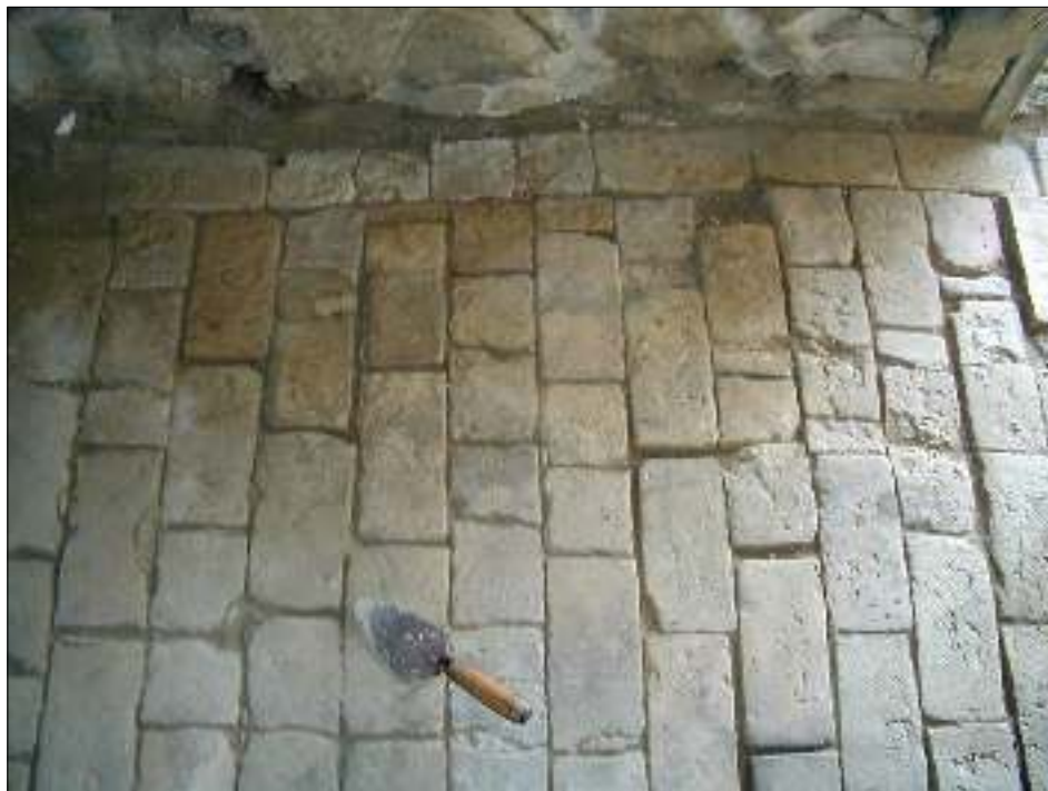
Figure 4-9. Brick floor prior to the excavation of Test Unit 3 in the Stone Cottage, 41SR311.
