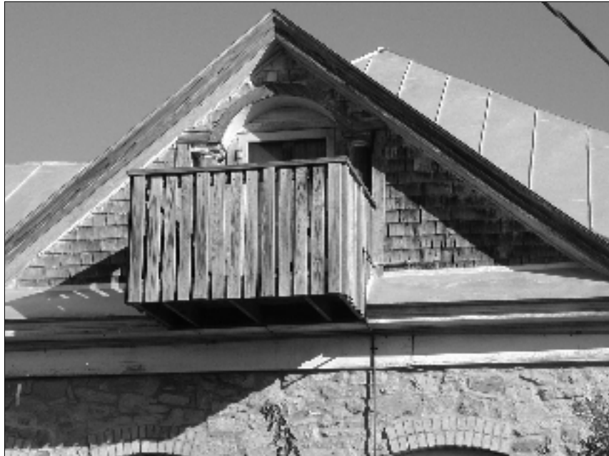
Figure 5-12. Detail of gabled roof and balcony, 41BX681.
