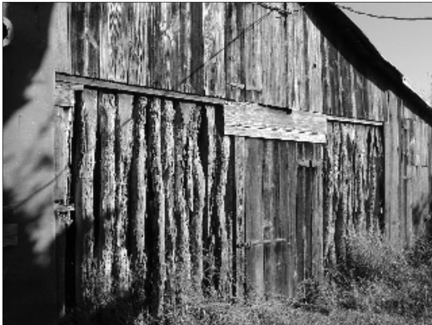
Figure 5-17. Construction detail of palisade barn, 41BX681.
