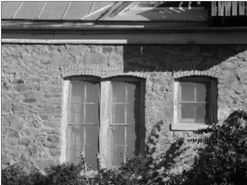
Figure 5-13. Window detail on east side of house, 41BX681.
