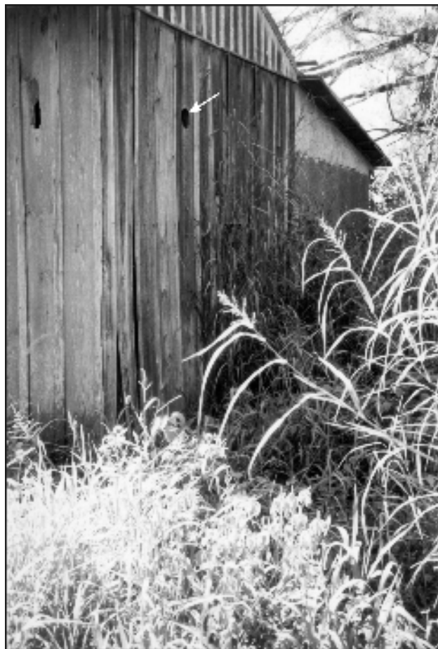
Figure 5-59. Stove pipe in west wall of structure at 41BX1575.
