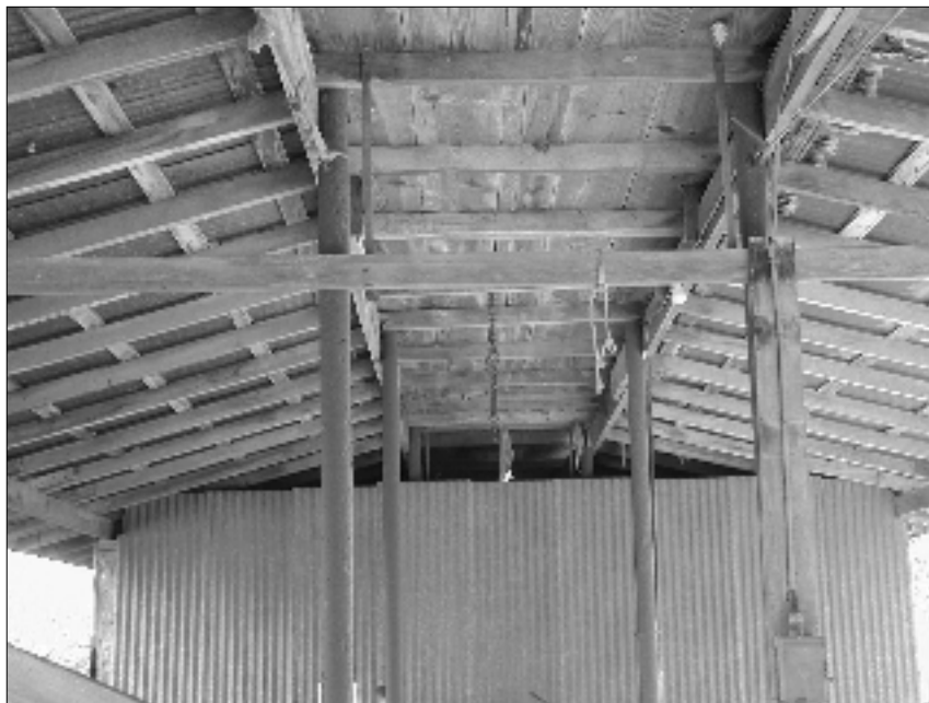
Figure 5-15. Detail of barn/stall roof, 41BX681.
