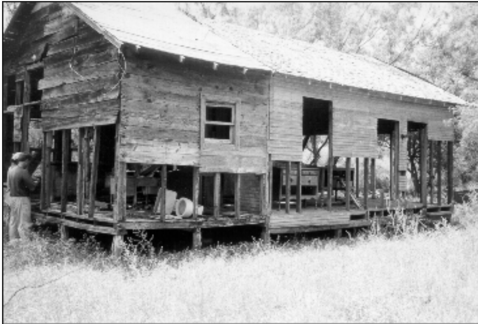
Figure 5-57. North wall of structure, 41BX1574.
