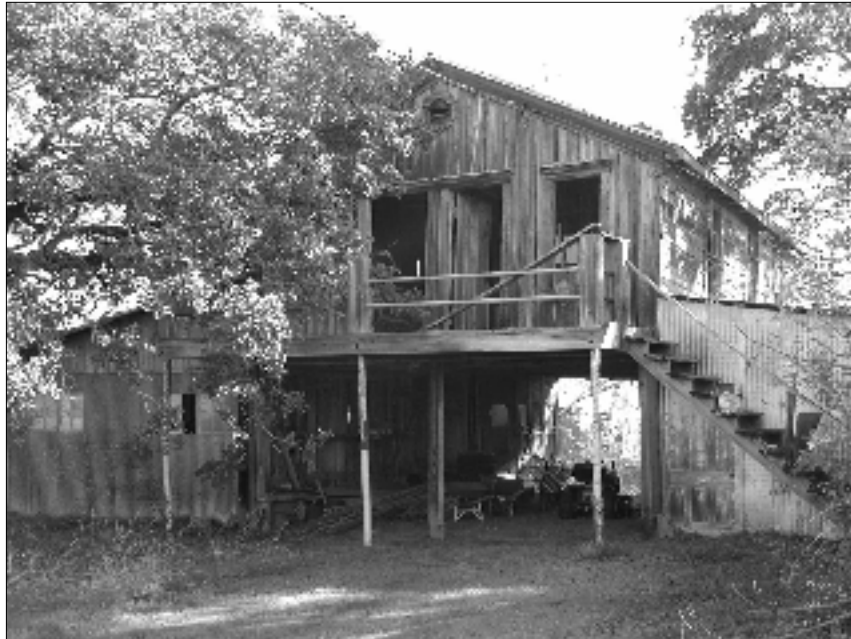
Figure 5-18. Barn-residence combination, 41BX681.
