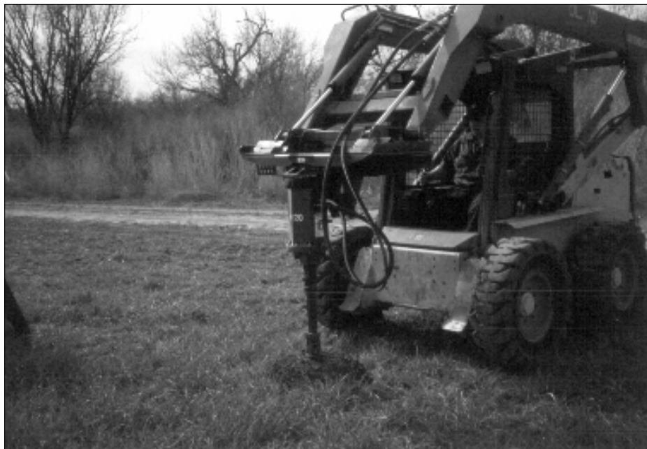
Figure 4-2. Mounted hydraulic auger used for auger testing.
