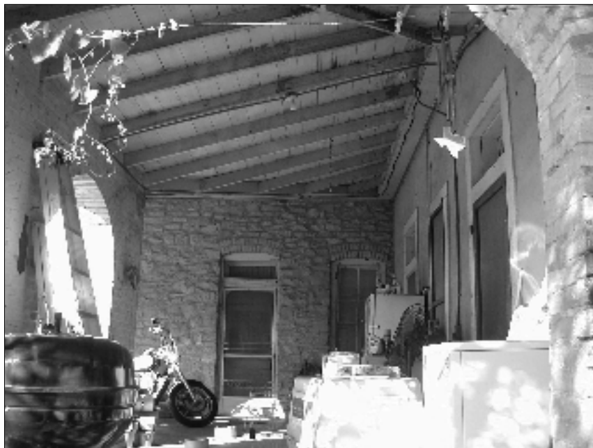
Figure 5-10. Interior view of porch at front of house, 41BX681.
