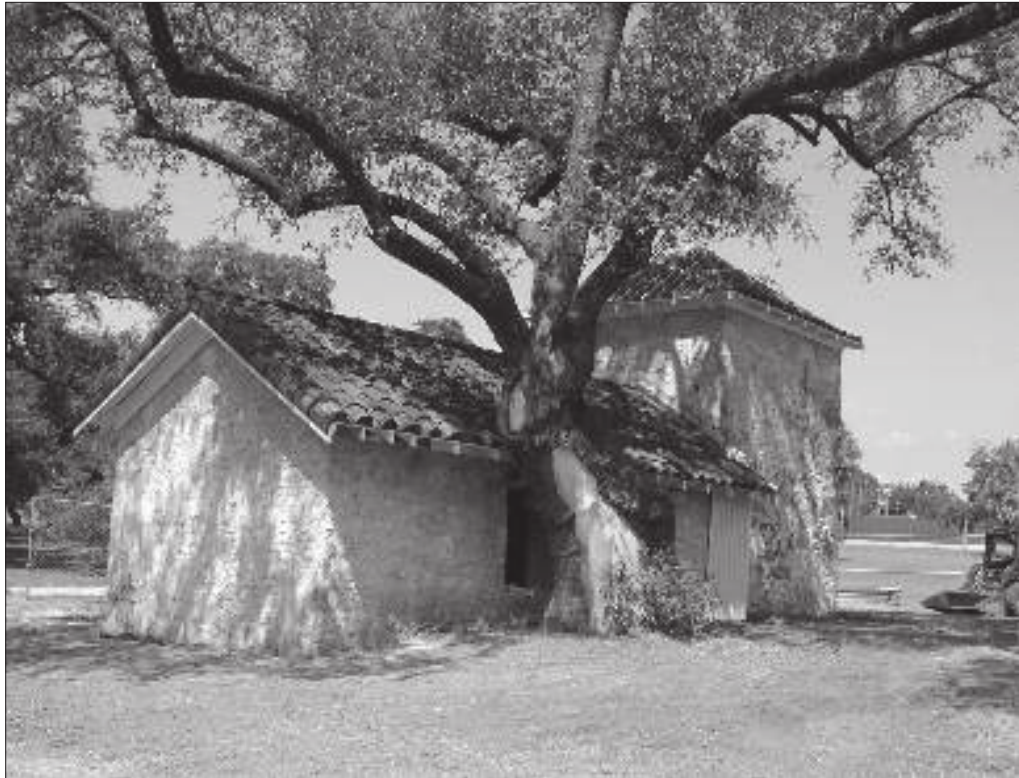
Figure 2. The Block House in 2002, during renovation.
