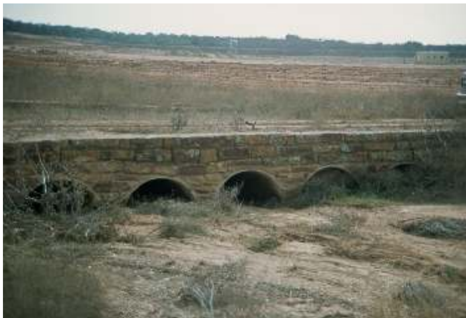
Figure 5. Bridge at site 41BR477. Photo by Alan Wormser, 1994.
