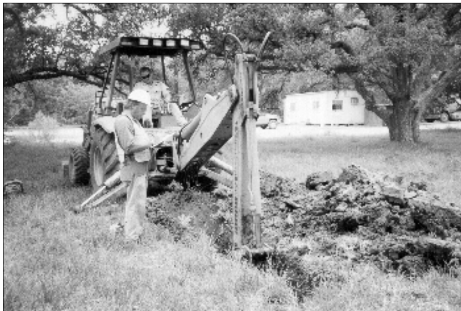
Figure 2-2. Typical lawn vegetation encountered along ROW.
