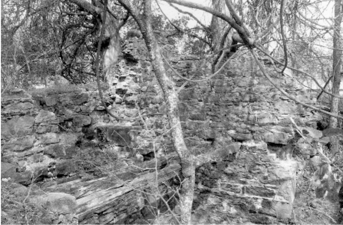
Figure 87. Aussilloux House showing remains of floor joists.
