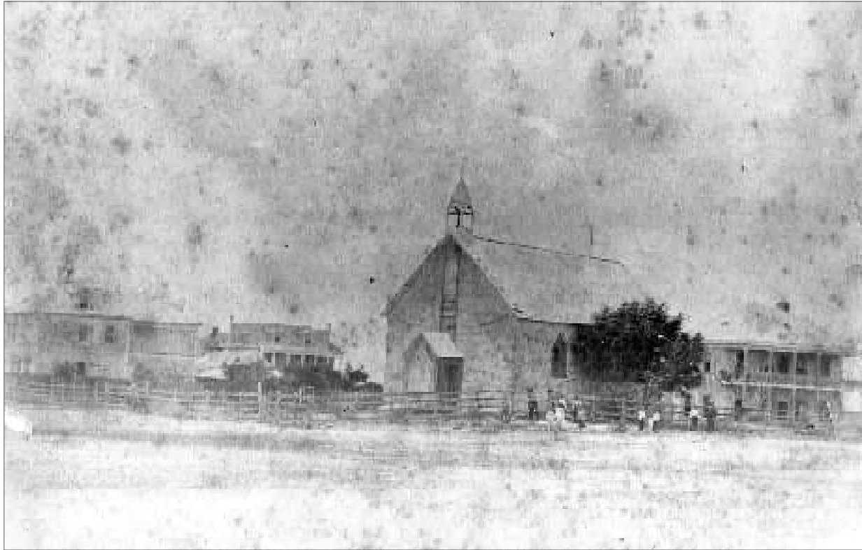
Figure 5-4. Our Lady of Refuge Church, ca. 1885, (left) Convent School, (right) Rectory, (background) Dolores Power Welder residence.
