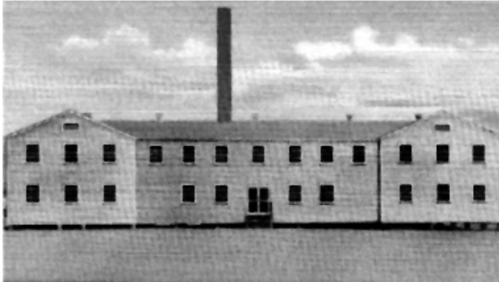
Figure 3-9. Division headquarters building, from Guide to the IRTC.
