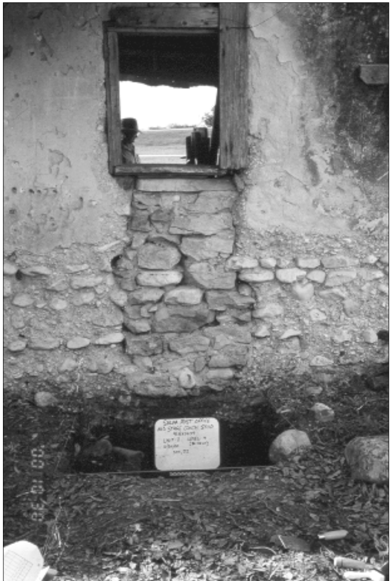
Figure 6. Location of Unit 2. Note repaired wall under window opening.
