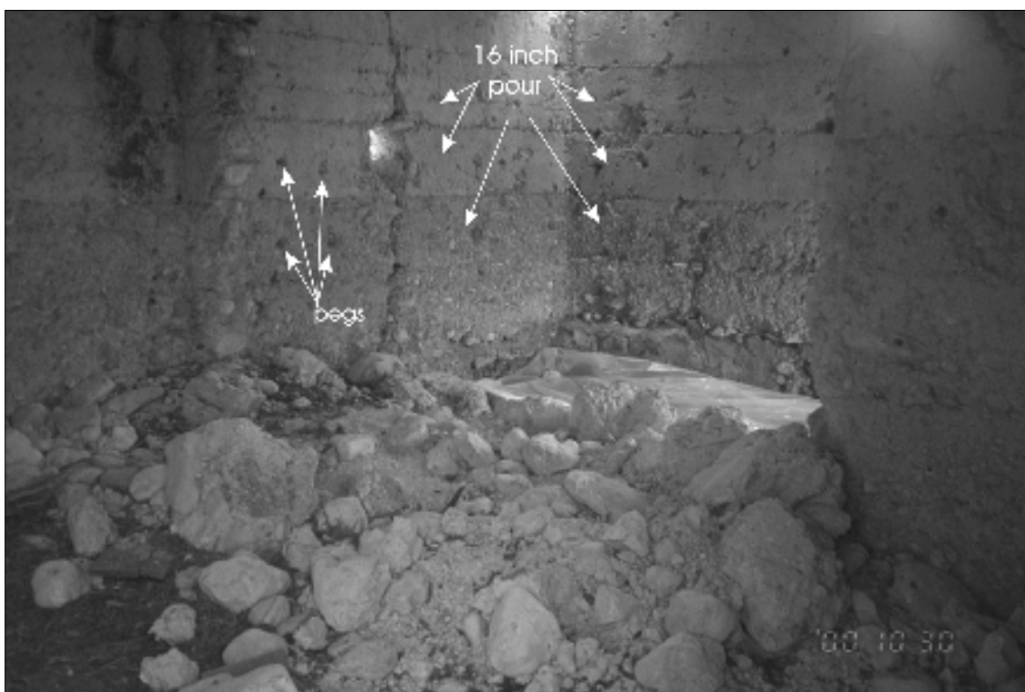
Figure 12. View of interior wall fall and tabby-related features (pours and pegs).
