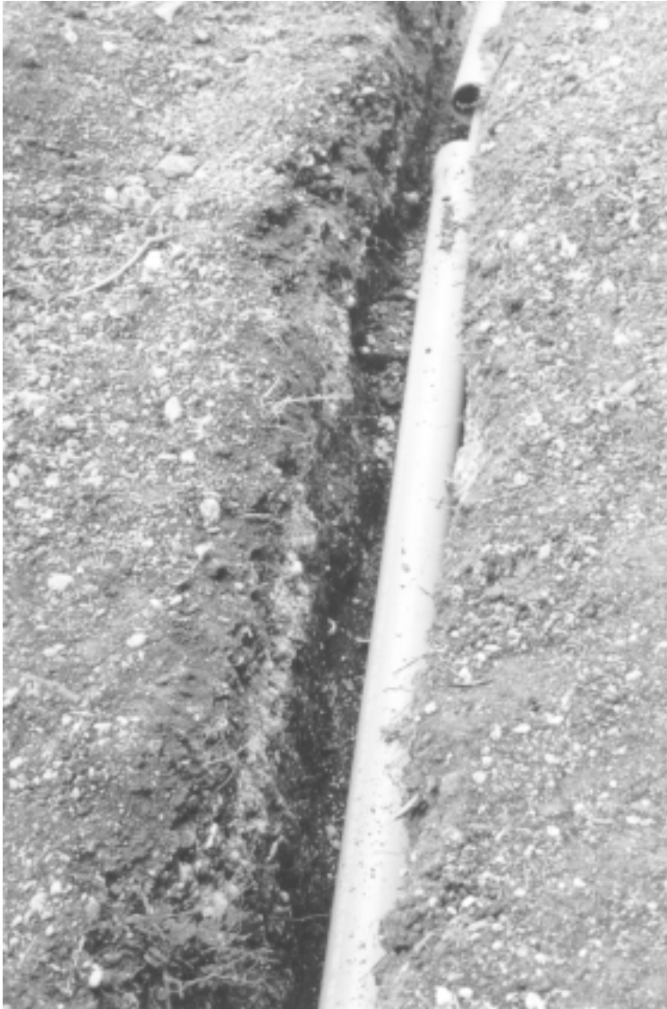
Figure 3. Electric line in 2-inch and 4-inch PVC conduit in Trench F.
