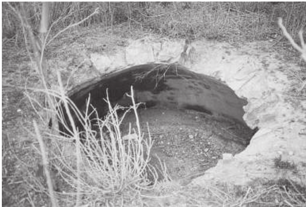
Figure 11-22. Cistern at the Keyes Dairy (41TG521).
