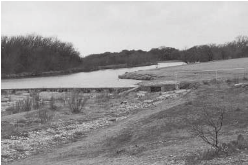
Figure 11-4. Photograph of White's Dam (41TG253) across Spring Creek, facing west, irrigation gate and ditch in foreground.
