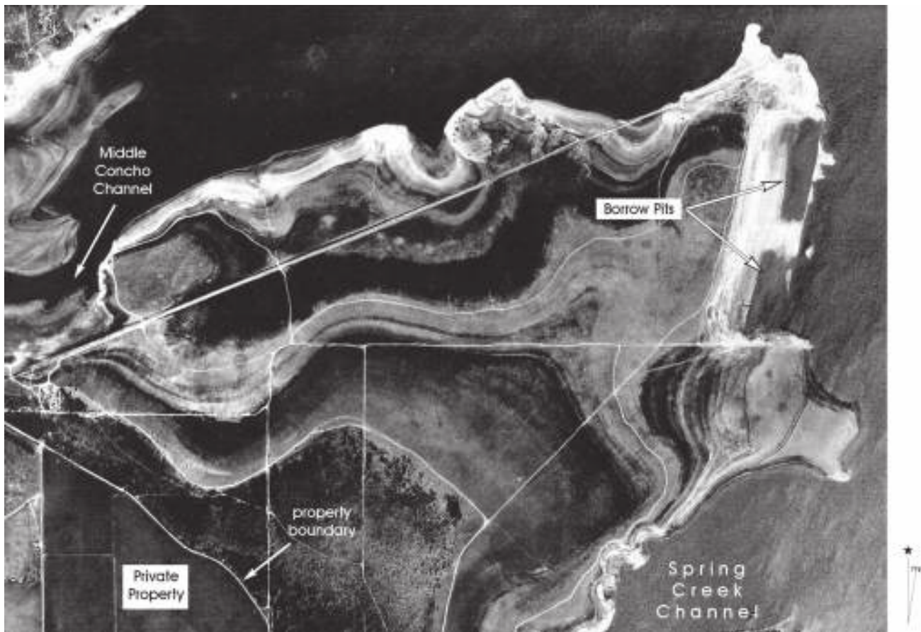
Figure 2-3. Enlargement of a USGS 1:10,000 color infrared aerial photo with borrow pits identified.
