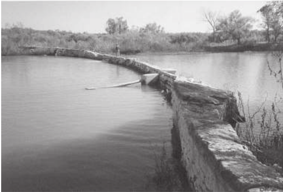
Figure 11-3. Photograph of Gardner's Dam (41TG248) across the South Concho River, facing southwest.
