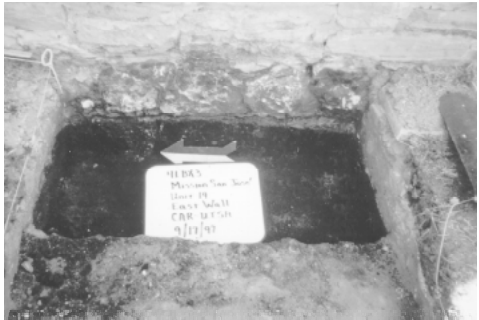
Figure 8. Base of east wall of southwest gate in Unit 19. Note that there is no underlying Colonial foundation beneath the CWA reconstructed wall.
