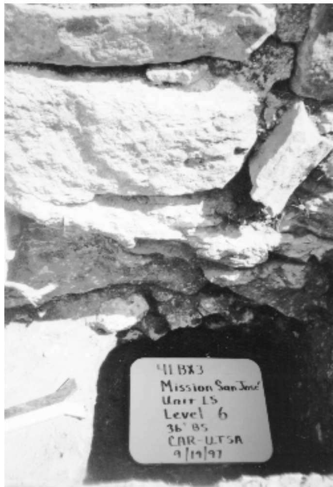
Figure 7. Large, blocky limestone on top of Colonial foundation and underlying the CWA wall in Unit 15.
