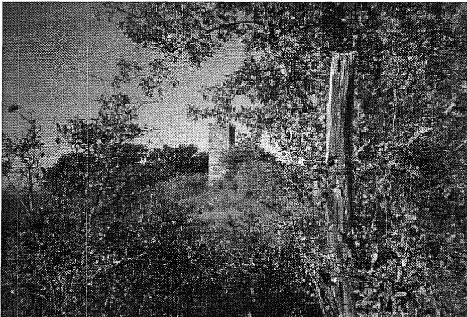
Figure 4. Photograph of the tower constructed by Colonel Coppock.
