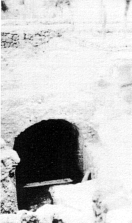
Figure 2. Vaulted turbine housing, facing south. Courtesy Daughters of the Republic of Texas Library.
