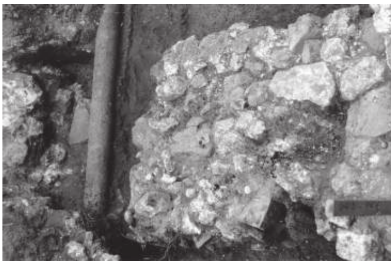
Figure 12. Exposed portion of interior wall foundation, top view.
