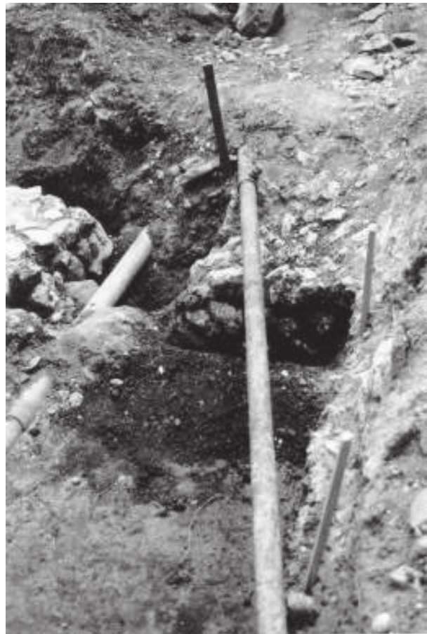
Figure 9. Exposed portion of the original exterior foundation. Looking south.
