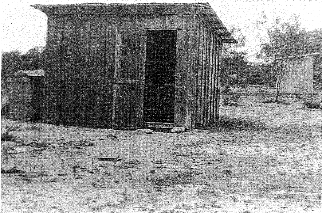
Figure 10-9. Delco generator house, ca. 1942, looking west. Laughlin AFB Base Properties files.
