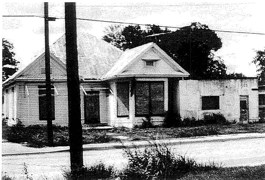
Figure 4-22. The Mendit Shop site.
