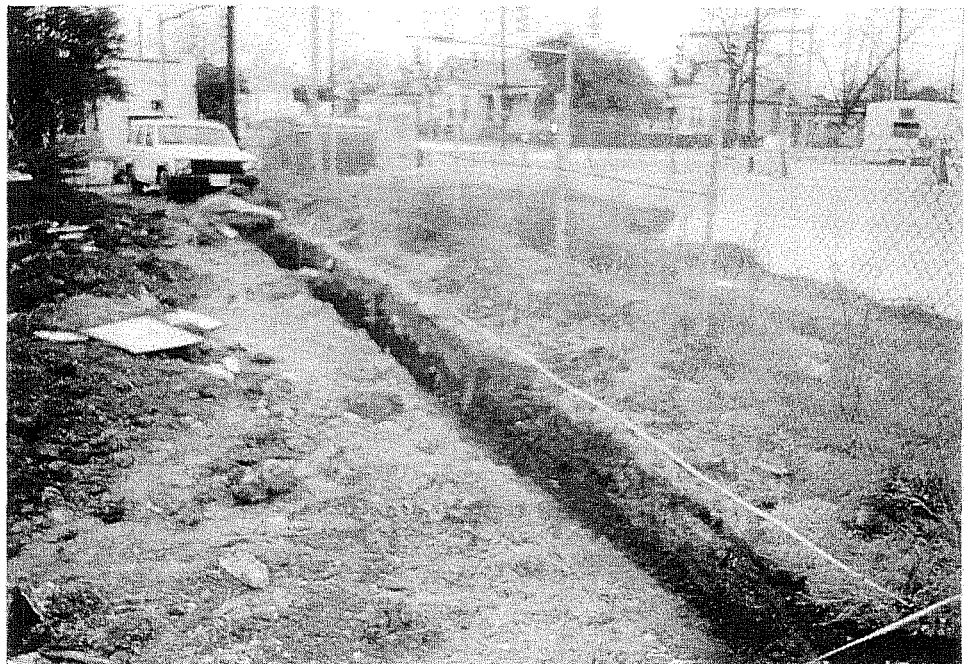
Figure 4-84. Trench E (Durango Street in background).
