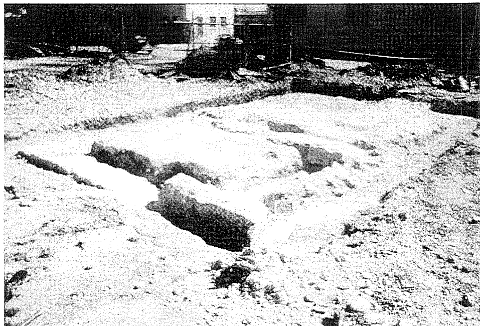
Figure 4-77. Foundation of the Gordon House.
