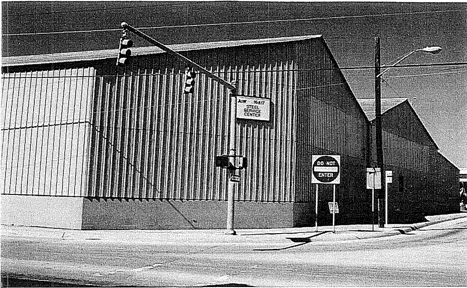
Figure 3-7. Steel Service Center, built during the 1960s.
