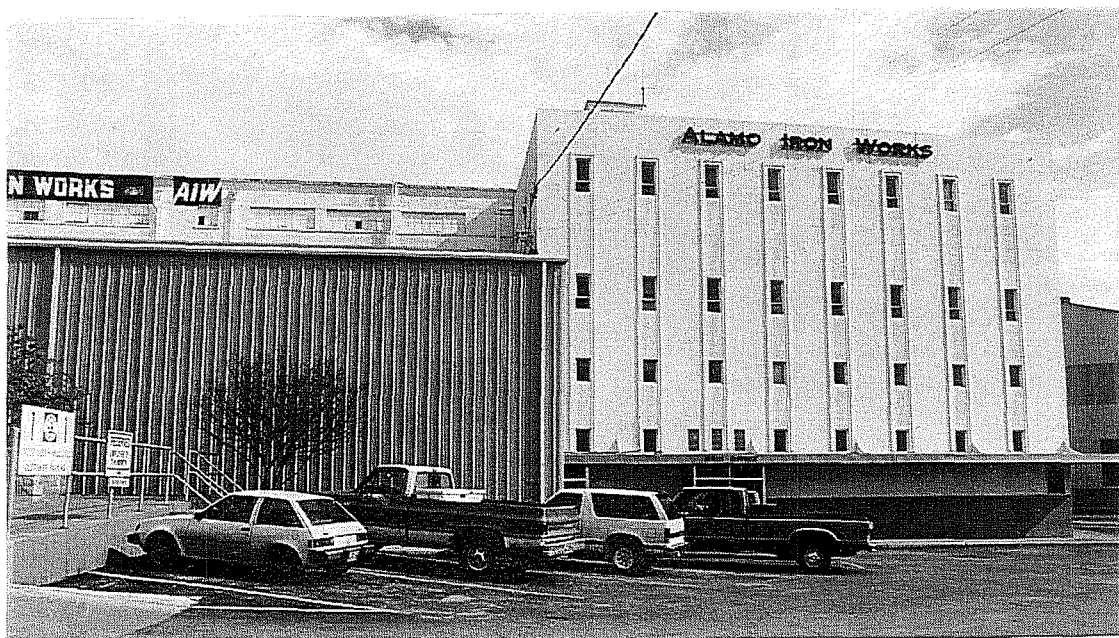
Figure 3-6. Alamo Iron Works, Corporate Office Building.
