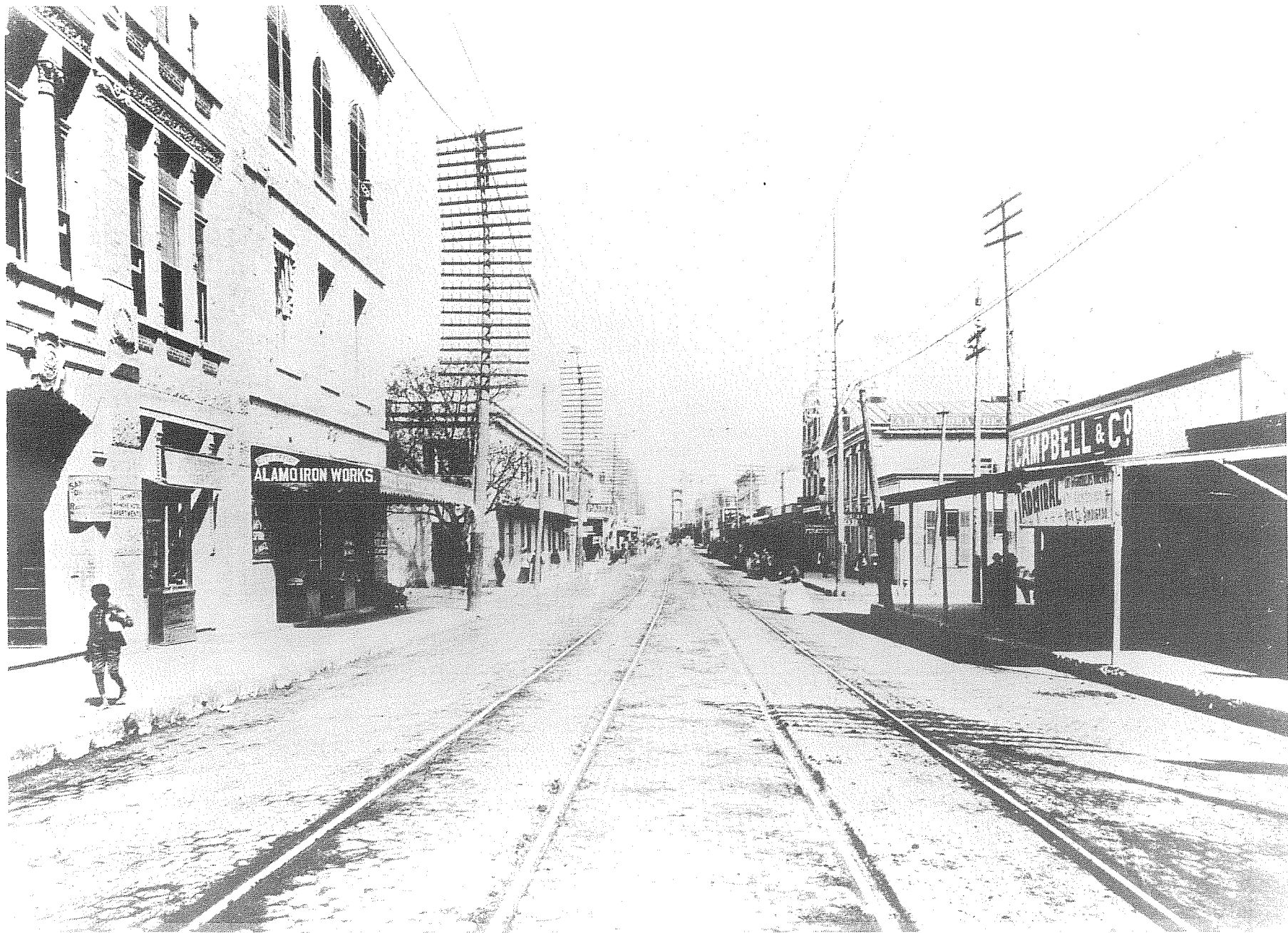
Figure 5. Houston Street, ca. 1900 . Looking east. Note the streetcar tracks and wooden pavers. Courtesy of the Daughters of the Republic Research Library, The Alamo.
