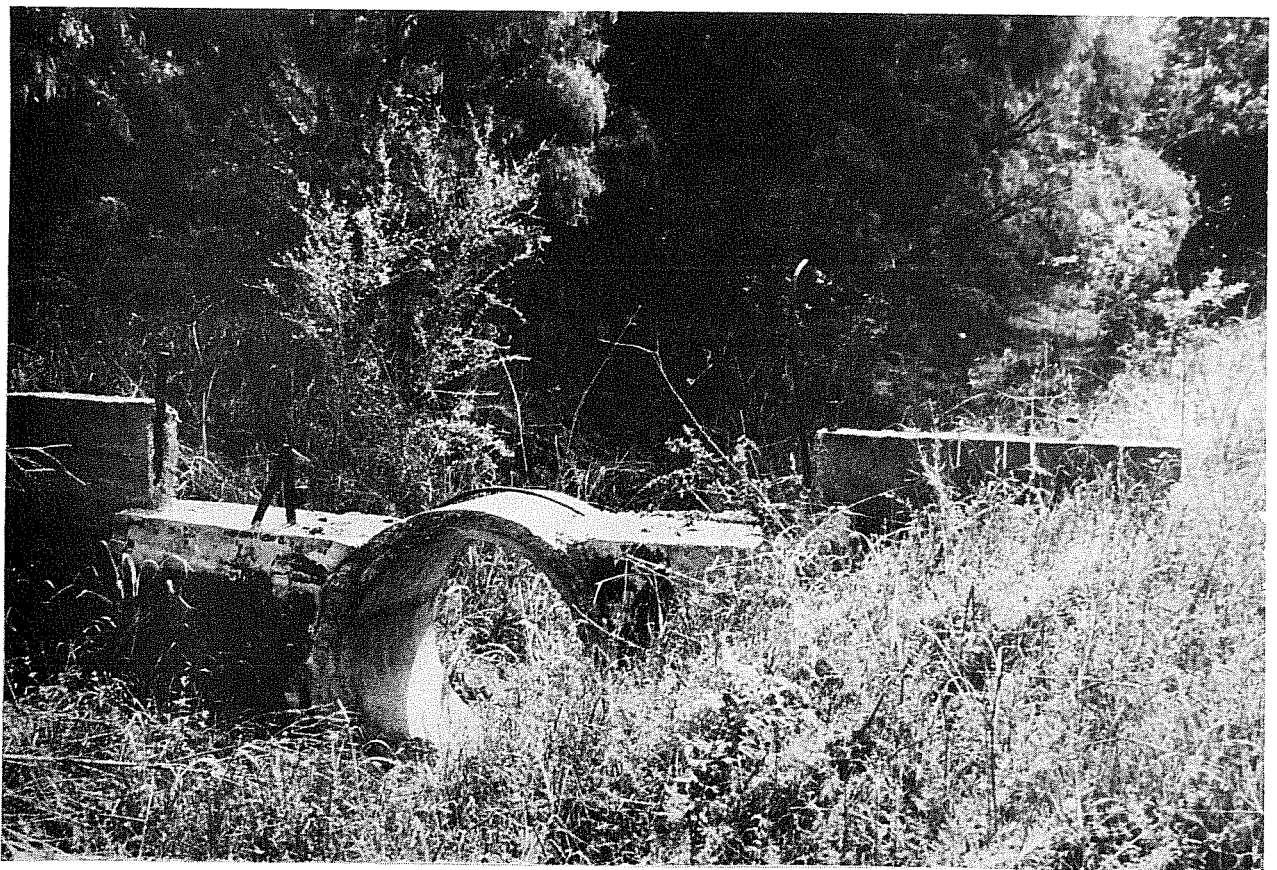
Figure 5. Views of Irrigation Near Confluence. a, irrigated fields northwest of Confluence site; b, early 20th century control gate in irrigation canal northwest of Confluence site.
